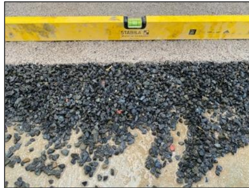
Figure H- 1: Screed layer placed on a core thickness of 20mm
