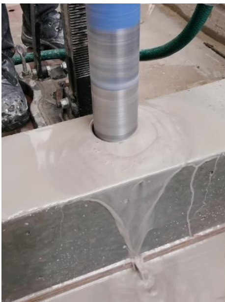
Figure 3.9 Beam being core-drilled, close-up
