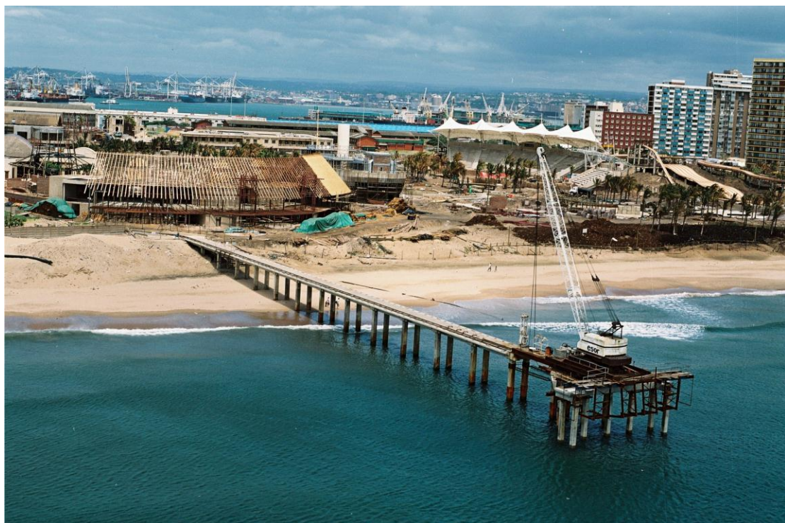
Figure 3.12: Construction of Jetty at Ushaka Marine World with the extra amount of purposed built jetty piles being constructed at the head of the Jetty.
