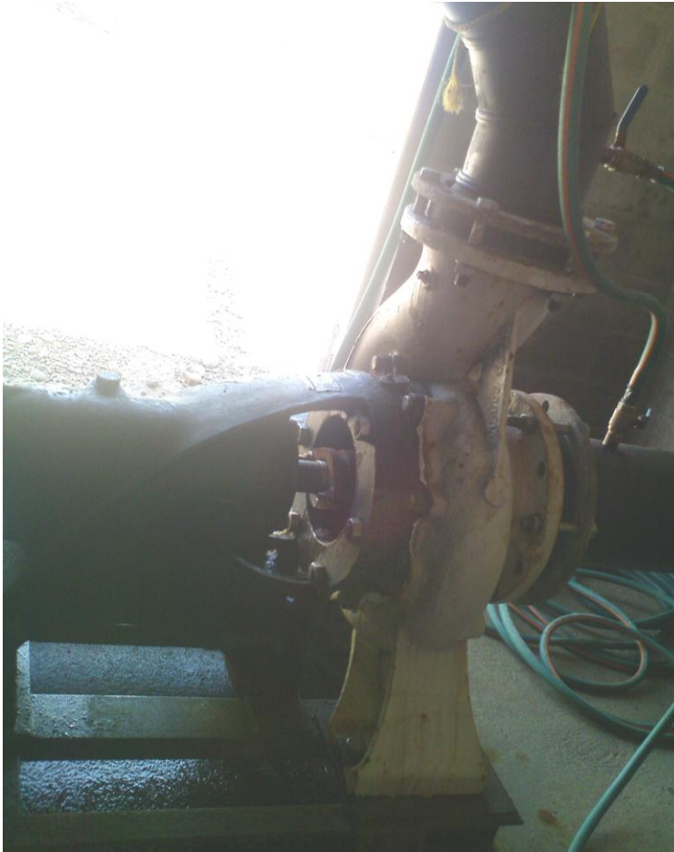
Figure 3.26: Centrifugal pumps, at Intake for West Coast Abalone
