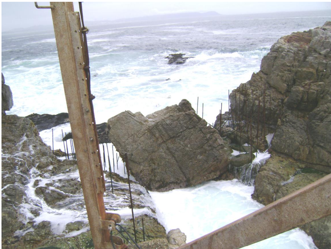
Figure 3.4: Strategically blasted rock placed at the entrance of the intake gully
