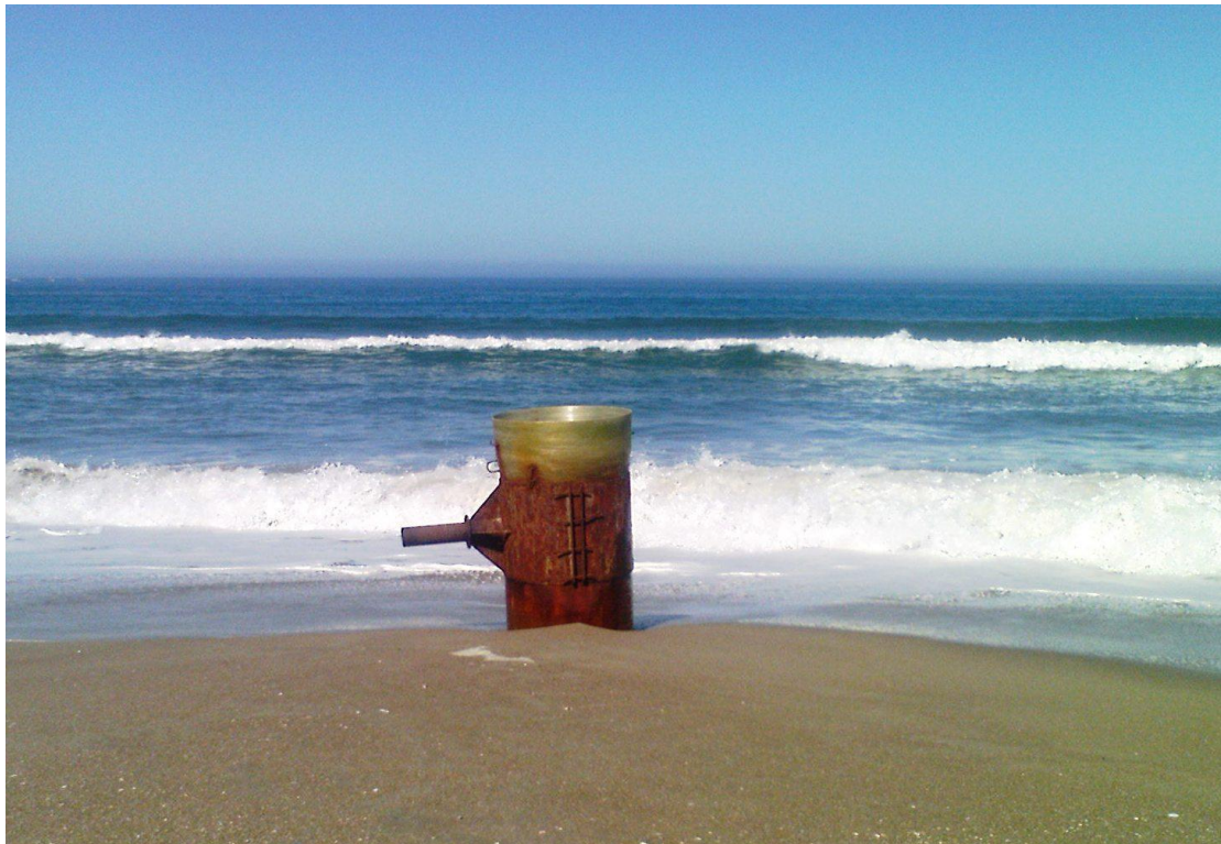
Figure 3.23: The metal sleeve with a bell end that has already been driven in to the sand
