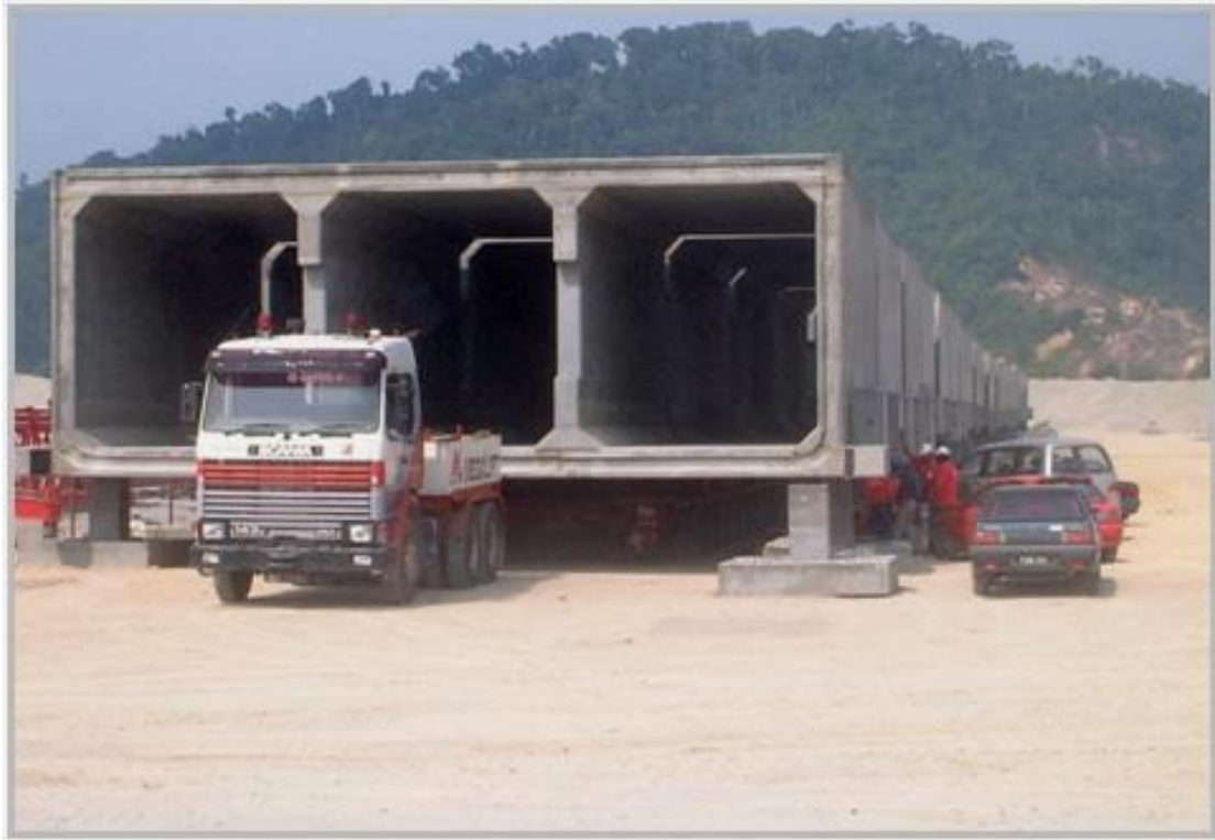
Figure 2.18: Majung Power Station seawater connecting culverts on land (ZLH, 2008a)
