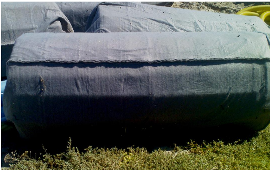
3.19: New Beach Well. Stitched geofabric covering the perforated intake pipe
