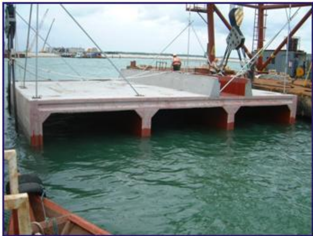
Figure 2.19: Majung Power Station seawater connecting culvert being floated and placed into position (ZLH, 2008a)
