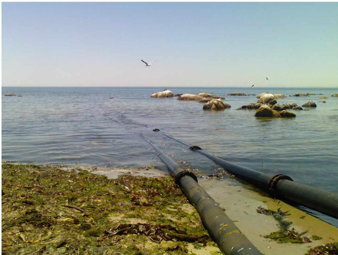
Figure 3.30: The intake pipelines for St Helena Abalone, 2No. \varnothing 300\text{mm} HDPE pipelines
