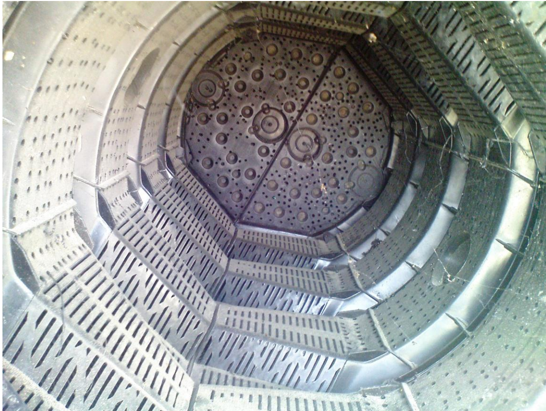
3.20: New Beach Well. Inside of the specially constructed perforated intake pipe
