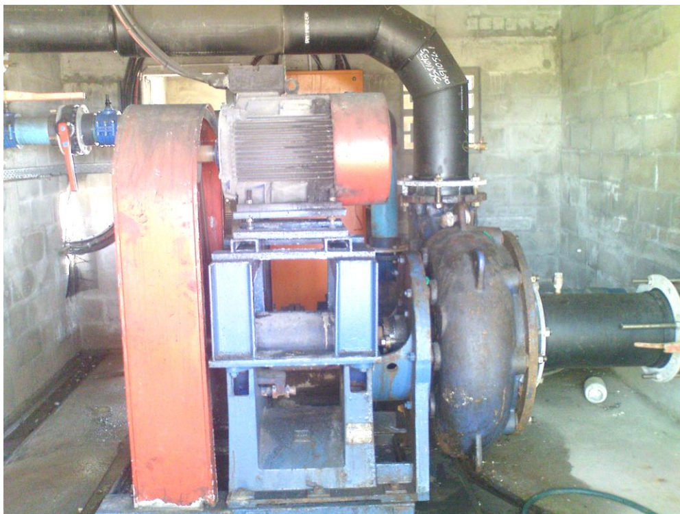
Figure 3.27: Slurry pumps, at Intake for West Coast Abalone
