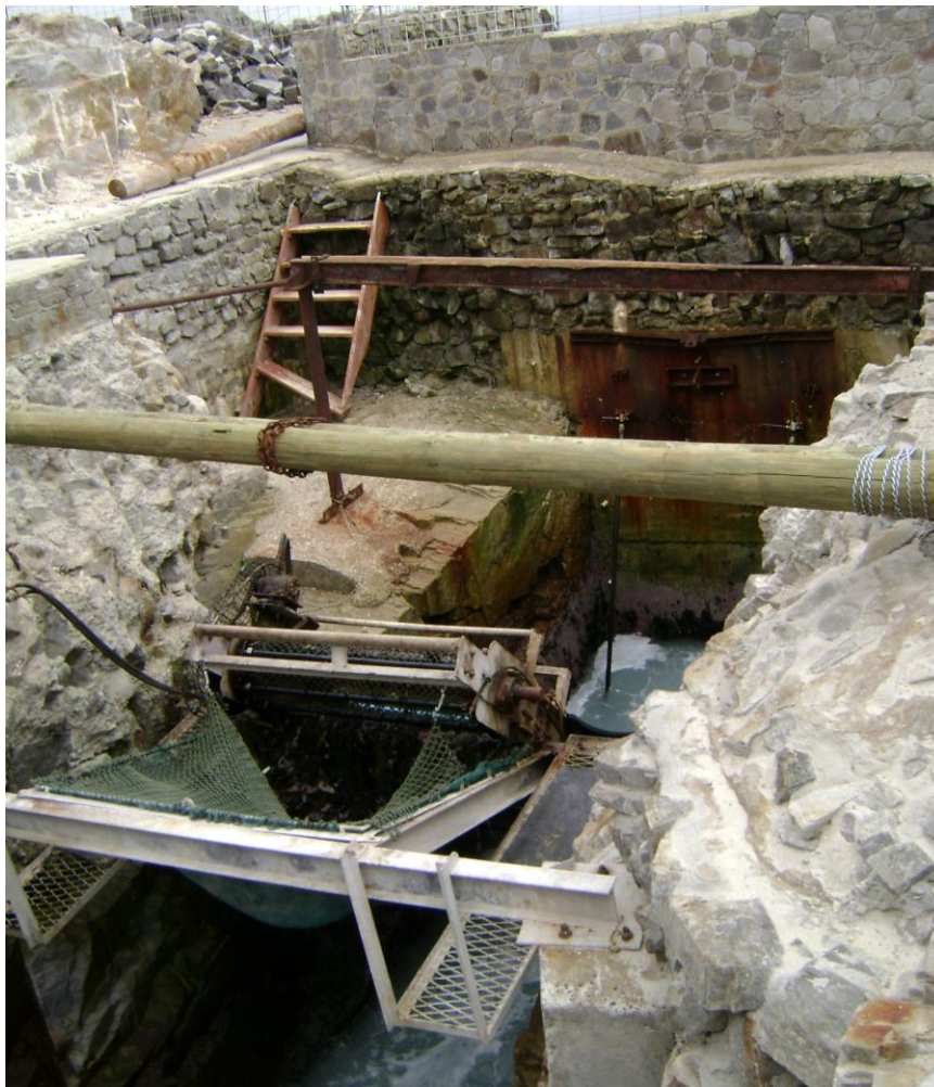
Figure 3.3: Looking seawards, the back end of the rotating screen can be seen in the foreground and the concrete screen wall in the rear
