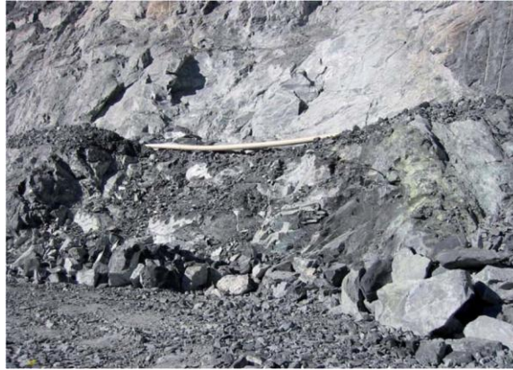
Figure 2.18: Location where the berm was lost (Geobrugg, 2008).
