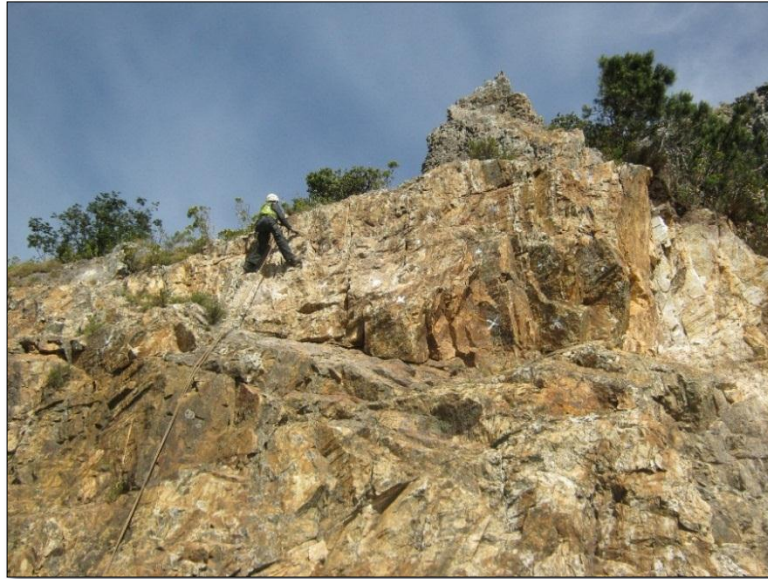
Figure 3.14: Area where the wedge was released and landed on the road, remaining wedge required stabilisation (Photo by S. Surujbally 2012).
