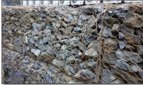
Slope side of Gabion Wall
