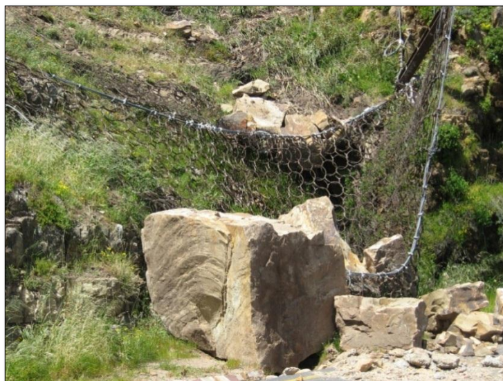
Figure 3.12: Large boulders breaching catch fence 15. (Photo by S. Surujbally 2007)
