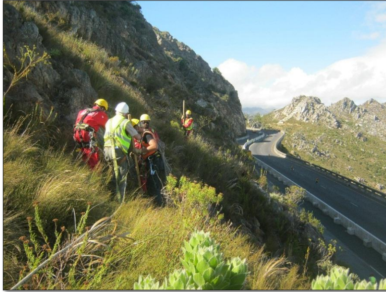
Figure 3.15 Visual inspection of the site and setting out of catch fence (Photo by S. Surujbally 2013).
