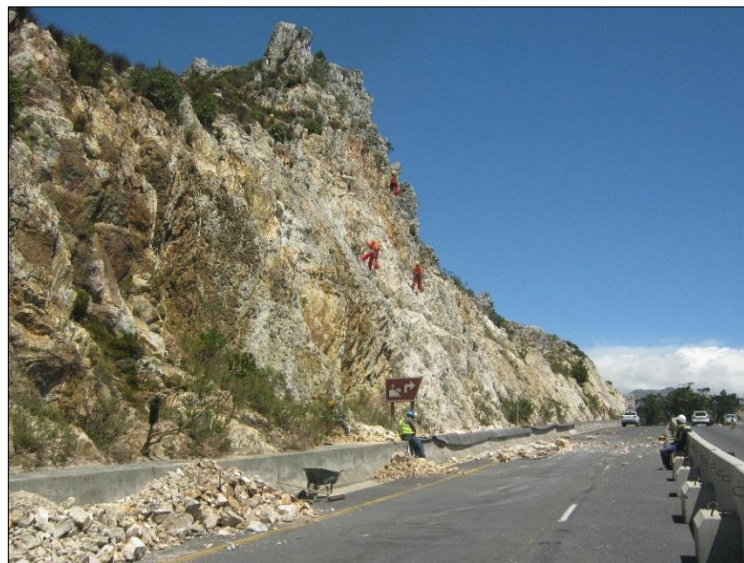
Figure 3.16: Barring down of loose rocks from the cutting face by rope access team (Photo by S. Surujbally 2012).
