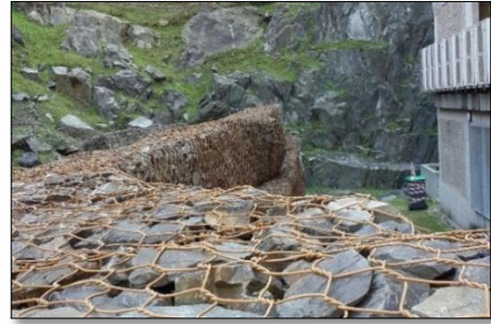
Gabion Wall bulging on the outside
