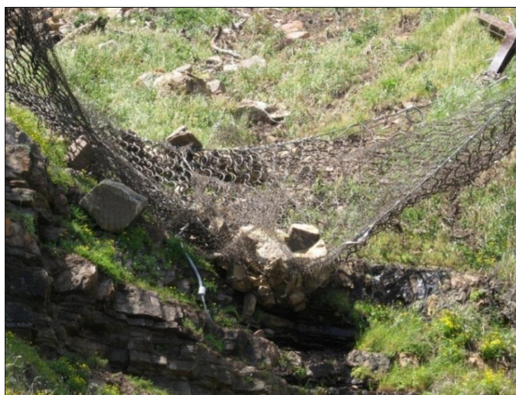
Figure 3.13 Multiple boulders breaching Catch Fence 15B (Photo by S. Surujbally 2007)
