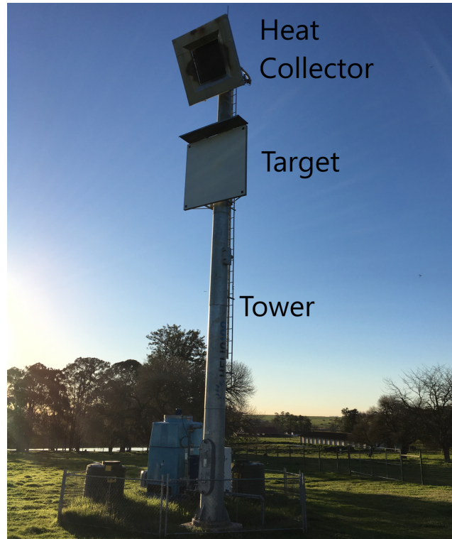
Figure 4.1: Helio100 central receiver
