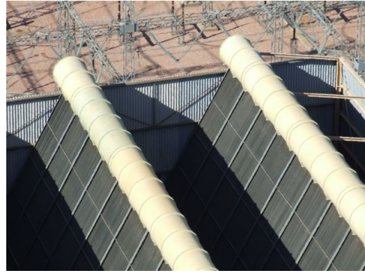
Figure 1.5: Steam ducts and inclined fin tube heat exchanger bundles
