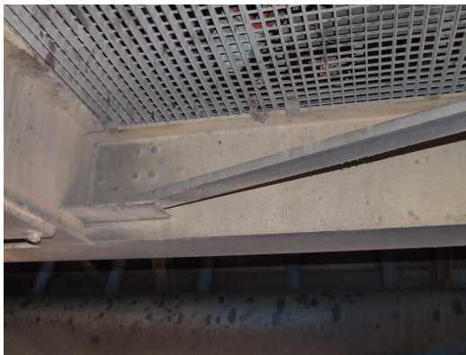
Figure A.5: Full-scale bridge from below showing walkway and I-beam construction
