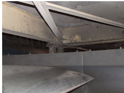
Figure A.6: Full-scale bridge from below showing I-beam construction and cross-members
