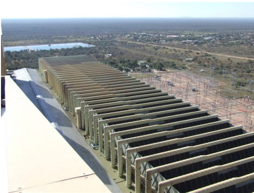
Figure 1.5: Steam ducts and inclined fin tube heat exchanger bundles
