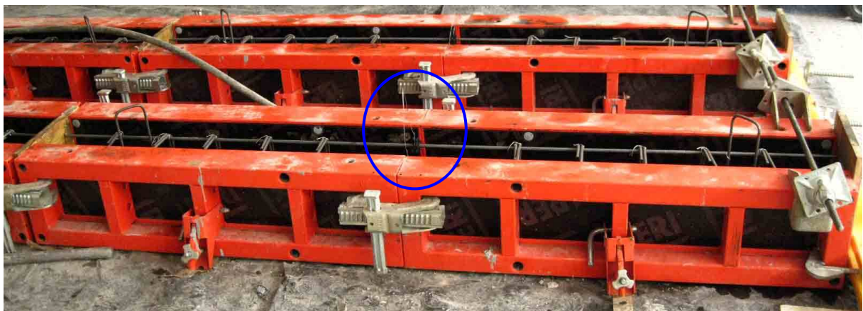
Figure 6.10: Reinforcing cages in the formwork.
