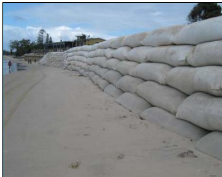
Figure 1-1: Kingscliff Seawall (Geofabrics Australasia Kingscliff Seawall Case Study, 2011)
