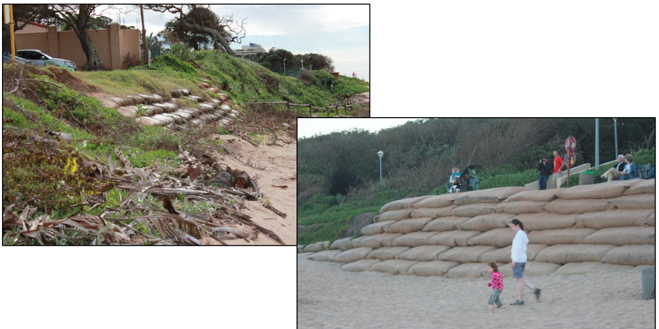
Figure 1-11: Photographs of GSC revetments at Umhlanga (Author, 2011)
