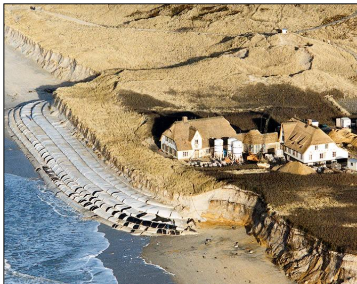
Figure 1-3: GSC Wrap-around Revetment in Sylt, Germany (Pianc, 2011)
