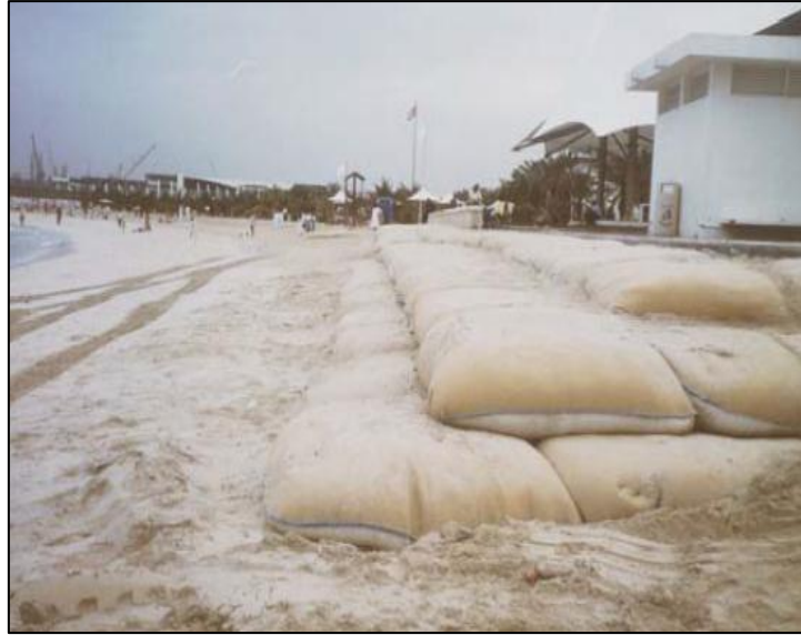
Figure 1-2: Jumeirah Open Beach (Geofabrics Australasia Jumeirah Beach Seawall Case Study, 2003)
