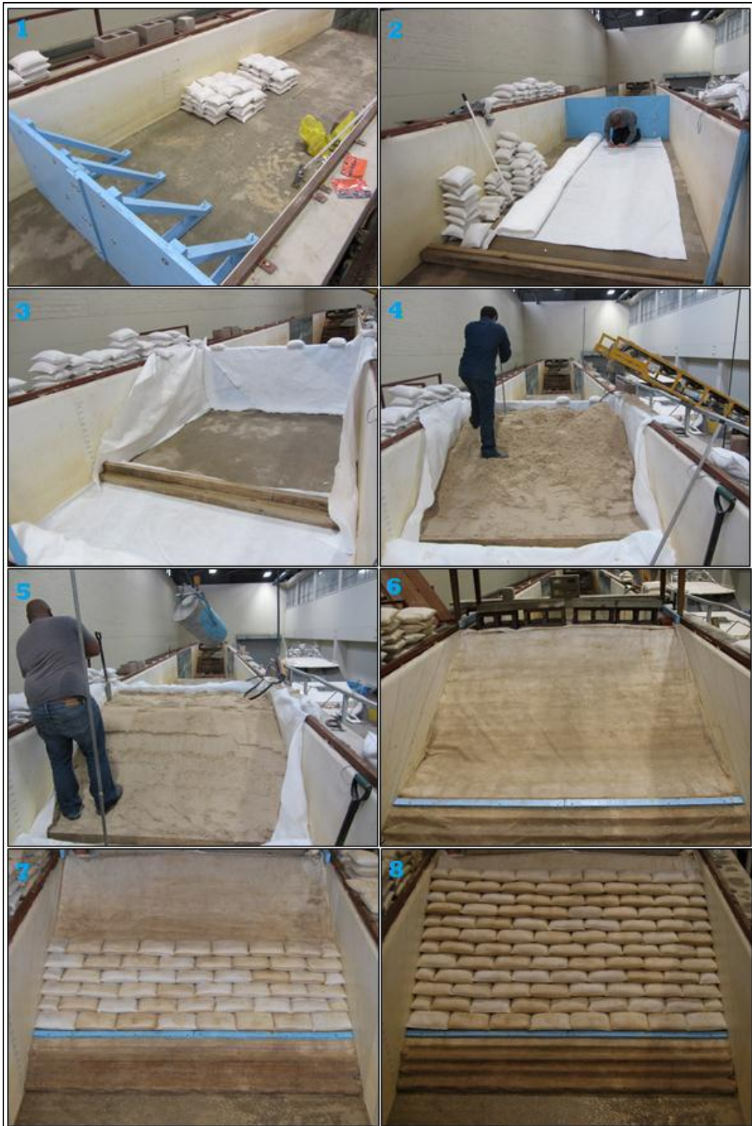
Figure 3-8: Photographs Showing the Construction of the Model GSC Revetment
