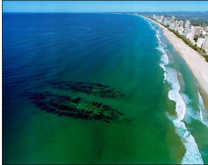
Figure 1-4: Artificial reef constructed of geotextile tubes. (Geofabrics Australasia Narrowneck Reef Case Study, 2000)
