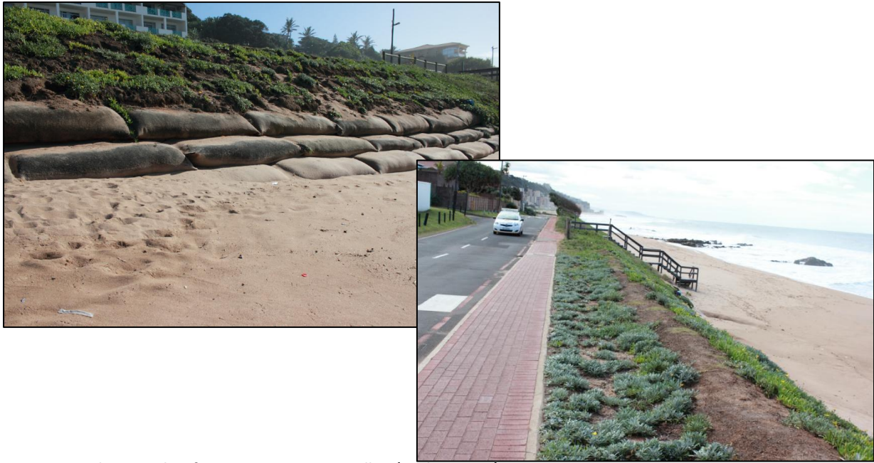
Figure 1-10: Photographs of GSC Revetment at Umdlotti (Author, 2011)
