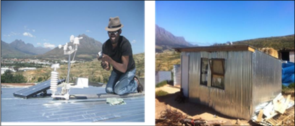
Figure 2: The iShack Project
