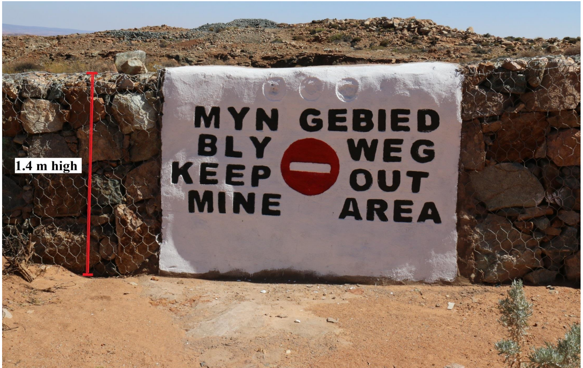
Figure 4. 2: The gabian wall surround the Rietberg Mine glory holes.
