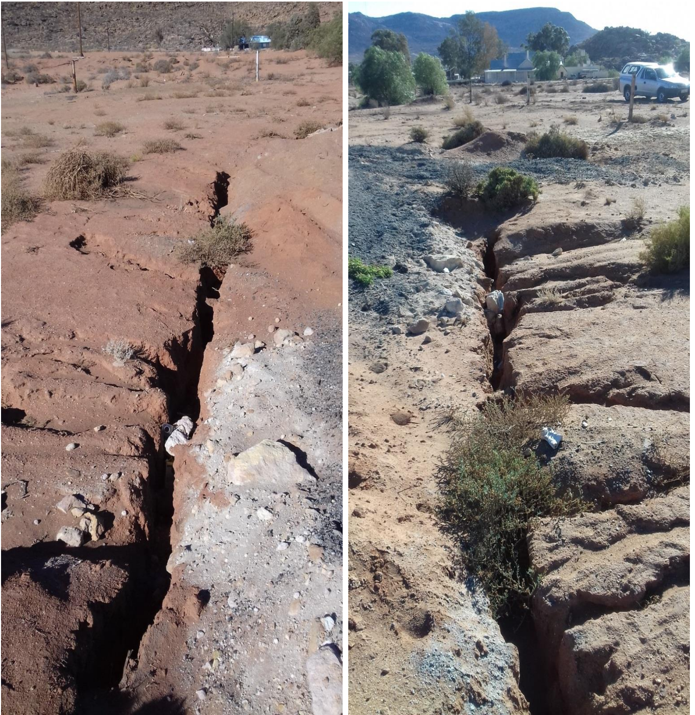
Figure 5. 11: The 15 cm-20 cm wide surface cracks outlining the gravel and sand filled East O'okiep glory hole.
