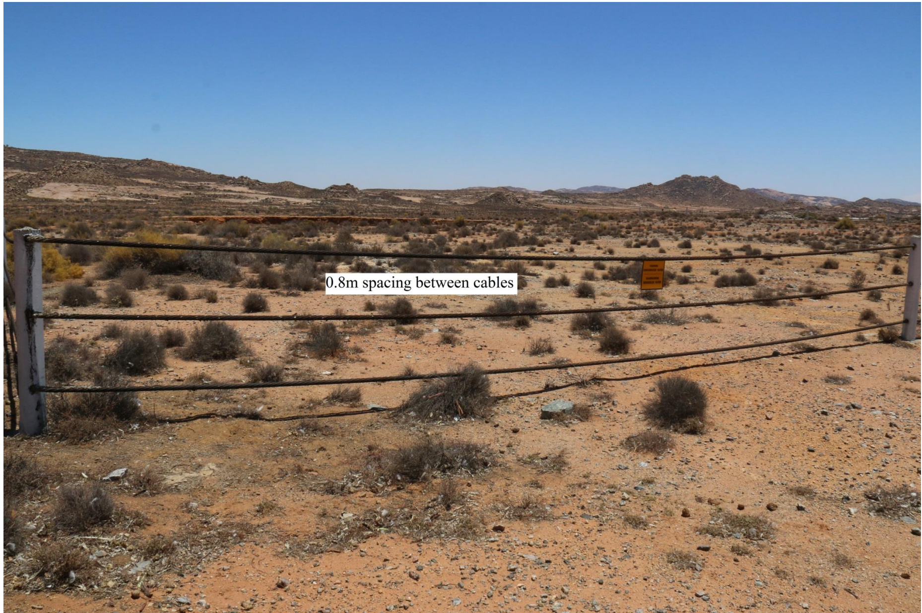
Figure 4. 13: The safety fence surrounding the Hoits Mine glory hole.
