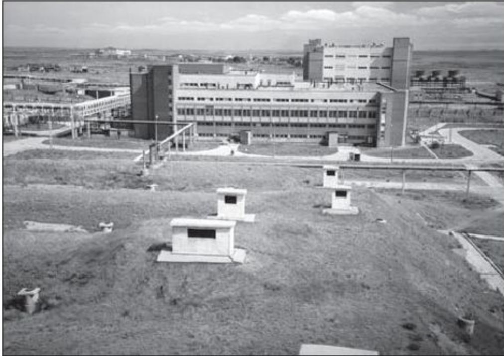
Photograph taken in 1995 showing three SNOB facilities: storage bunkers in foreground, Building 211 behind bunkers, and Building 221 in background. (Photographer: Andrew C. Weber.)
