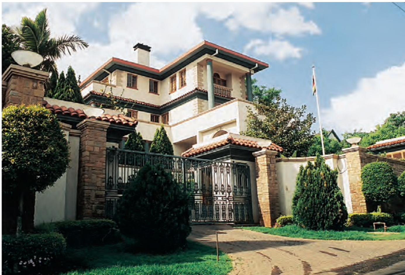
Figure 45: Basson was involved in the refurbishment of Merton House, in Arcadia, Pretoria, at a cost of R10 million. The property was later sold to the Zimbabwean government for R7,5 million and continues to serve as an embassy. (Burger & Gould, 2002).
