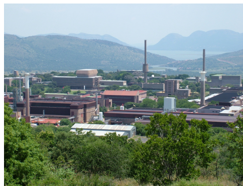
(b) The Pelindaba site, home to the SAFARI-1 reactor [146]
