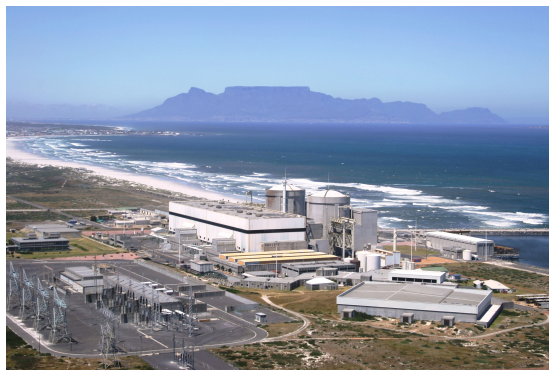
(a) The Koeberg Nuclear Power Station [161]
