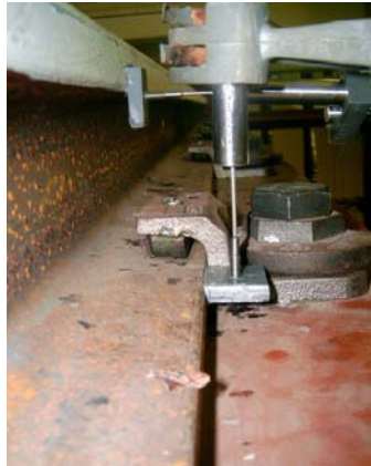
Photo 6.4: LVDT's measuring deflection of girders
