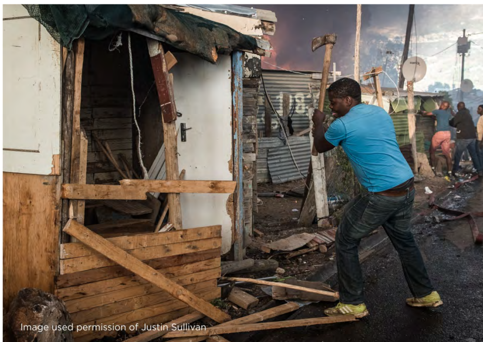
Figure 6-8: Dry firefighting techniques being employed by a resident trying to demolish his home to prevent spread and possibly save the construction materials. (Image used permission of Justin Sullivan)
