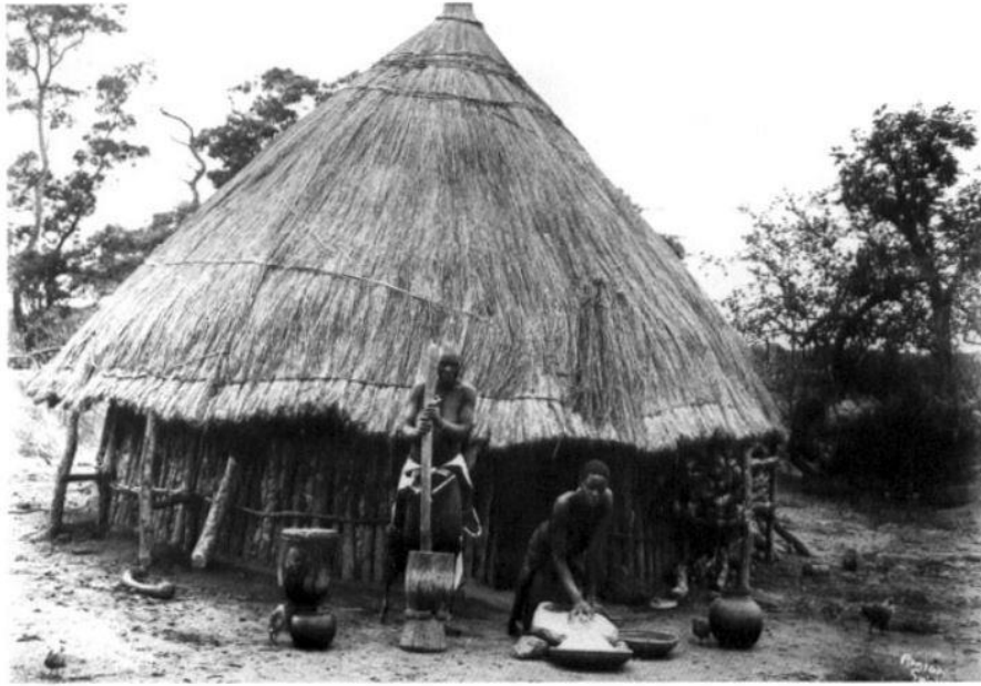
Figure 2: Typical traditional Shona homes occupied from around the 1850s onwards. 65
