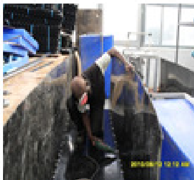
Construction of 3meter Biofilter
