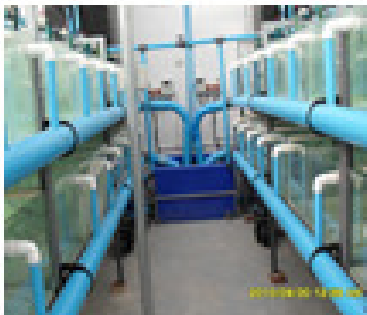
Completed system with pumps, sumps, biofilter & glass tanks
