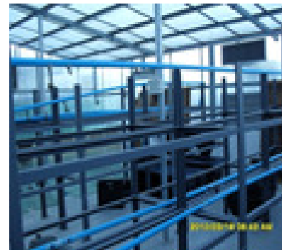
Steel Platforms that will hold the glass tanks
