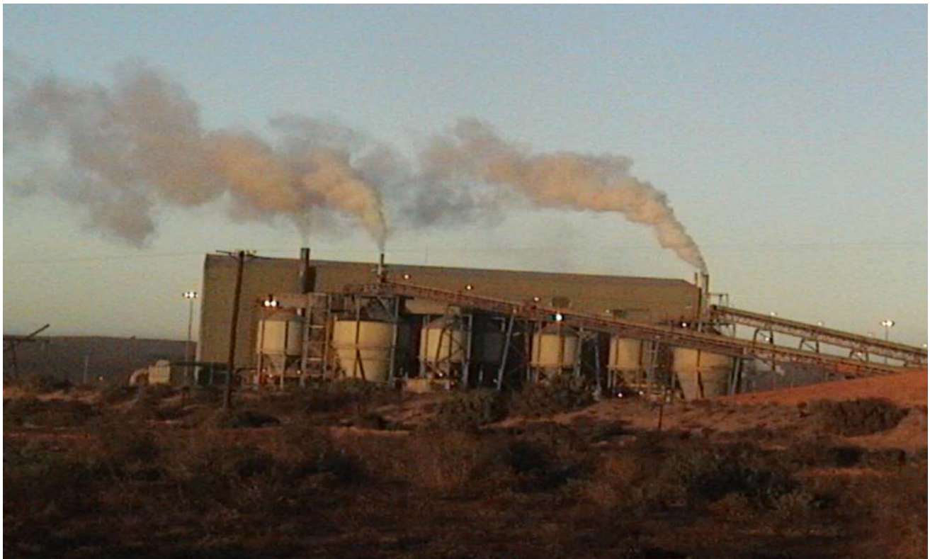
Figure 2.1: The release of acid emissions into the atmosphere from the stacks at the Mineral Separation Plant. The gaseous emissions are driven inland or east wards by the prevailing westerly winds.
