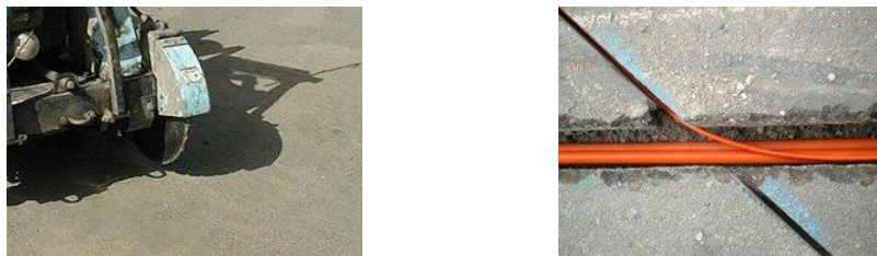
Figure 71: Constructing a micro duct system
