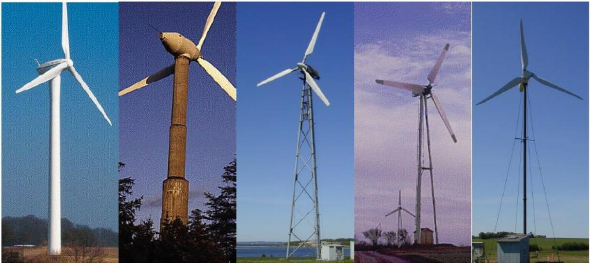
**Figure 2.8:** Various types of HAWT tower structures
