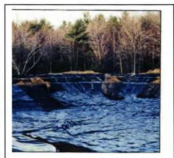
Figure 5.3 Installation of a HDPE liner in earthen ponds (AquaticEco catalogue 2003)
