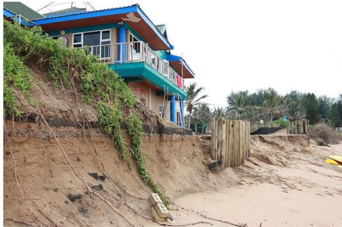
Figure 4.37 Erosion of the Alkantstrand Beach threatening the lifeguard house (Zululand Observer, 2014)
