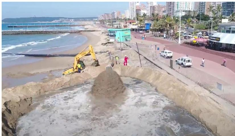
Figure 3.24 Example of beach nourishment along a groyne field in Durban (extracted from video by TNPA, 2018)
