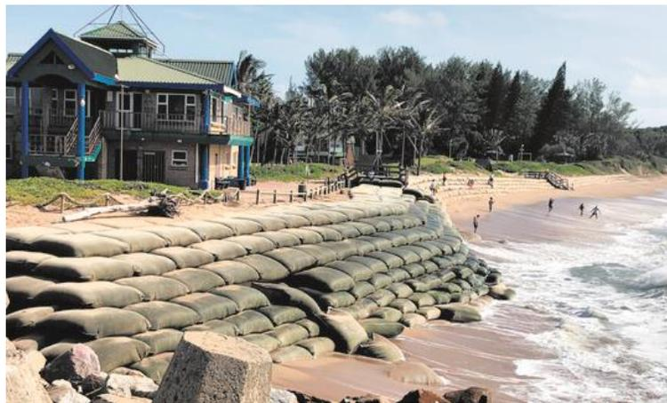
Figure 4.38 Geotextile bags slipping compromising the defence (Zululand Observer, 2021)
