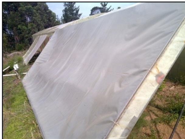
**Figure 19 Solar water heater panels**
