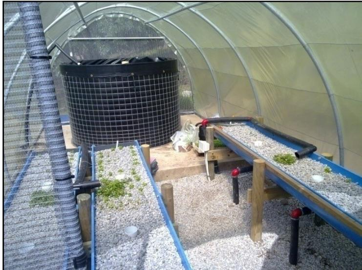
Figure 33 Section of system 6 enclosed in greenhouse showing a tank and growbeds
