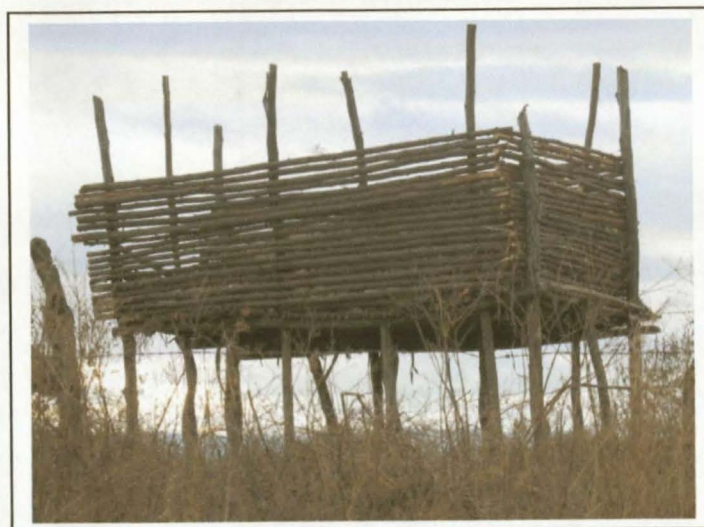
Figure 5: A picture showing the traditional maize crib at Maphalaleni in the Highveld. It was elevated so that livestock could not reach the stored crop. There is no roof. This maize crib however was built using nails.
