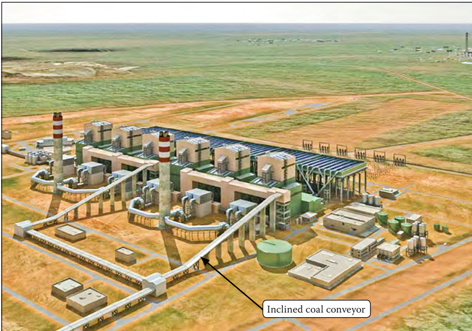
Figure 1 Medupi Power Station (Source: Eskom)
