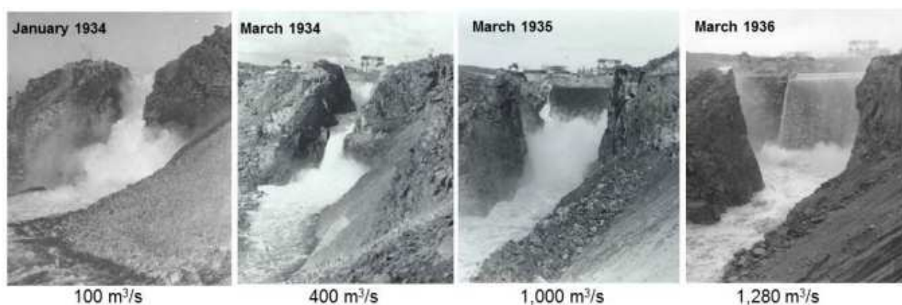
Figure 2-20 - Scour progression of Ricobayo Dam for the different discharges [56]
