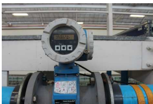
Figure 4-4 - Electromagnetic flow meter
