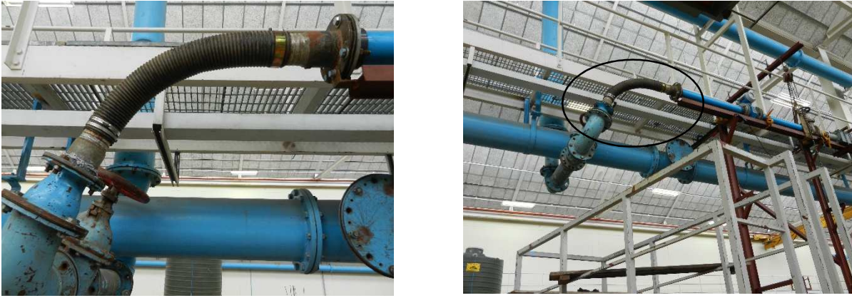
Figure 6-17 - Bended pipe connection at issuance
