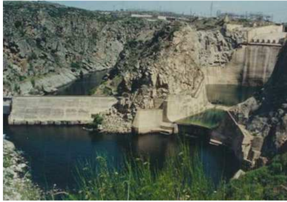
Figure 2-21 - Scour remediation of Ricobayo Dam [56]
