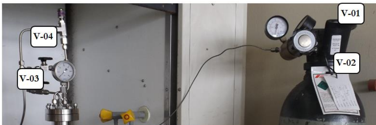
Figure B.1: Valves used for pressurisation and depressurisation procedures
