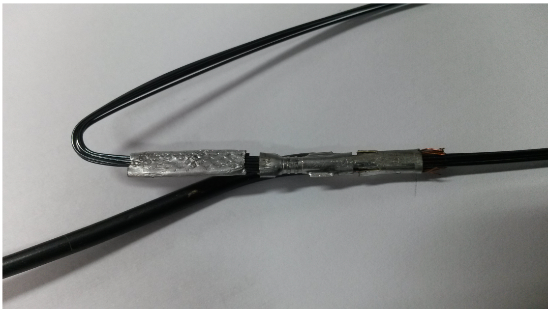
FIGURE 6.28: Partial view of bundle construction(Crimping)
