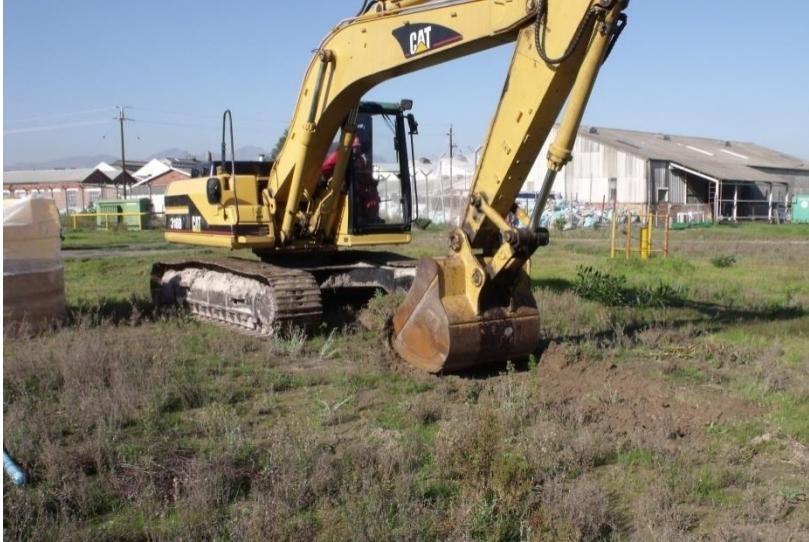
Figure 34: Excavator used for digging to below the water table.
