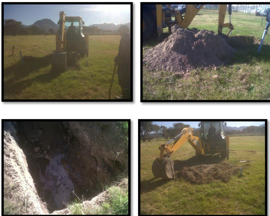
Figure 44: Excavation to the depth at the top of the tank for sampling of the woodchips within the tank.
