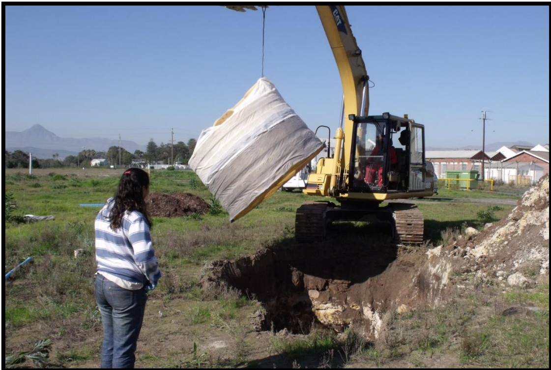
Figure 40: Lowering of the tank into the excavated area prior to filling and compacting of woodchips
