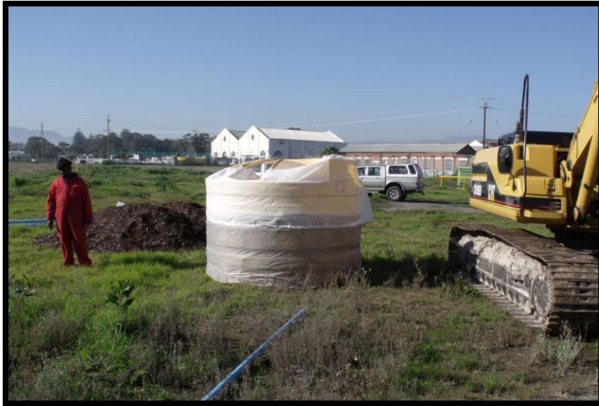
Figure 36: Biddum cloth placed around the tank to prevent larger grain sizes from clogging slits along the circumference of the tank
