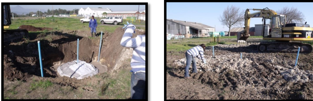
Figure 43: Filling of the excavated area, the picture on the left shows the groundwater that had already seeped into the tank while the emplacement and filling was taking place.
