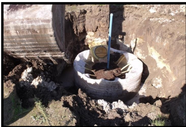
Figure 42: Filling and compacting of the woodchips in the tank
