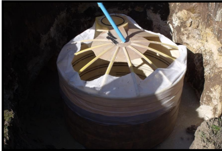
Figure 41: Central monitoring point inserted into the circular opening in the tank
