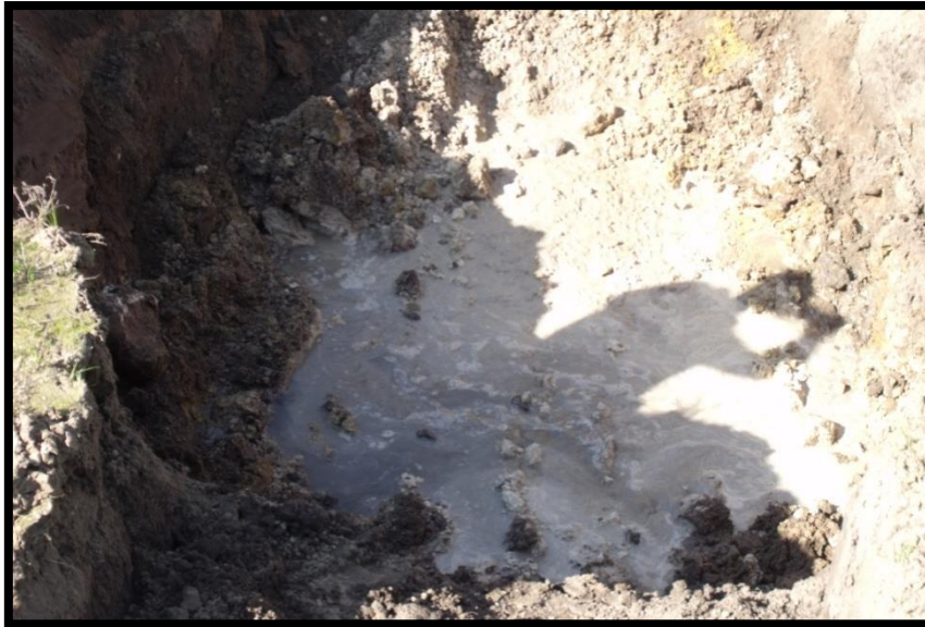
Figure 38: Resultant visual after reaching the water table. Water seeped from the side walls of the excavation at approximately 1.35 m below surface level.
