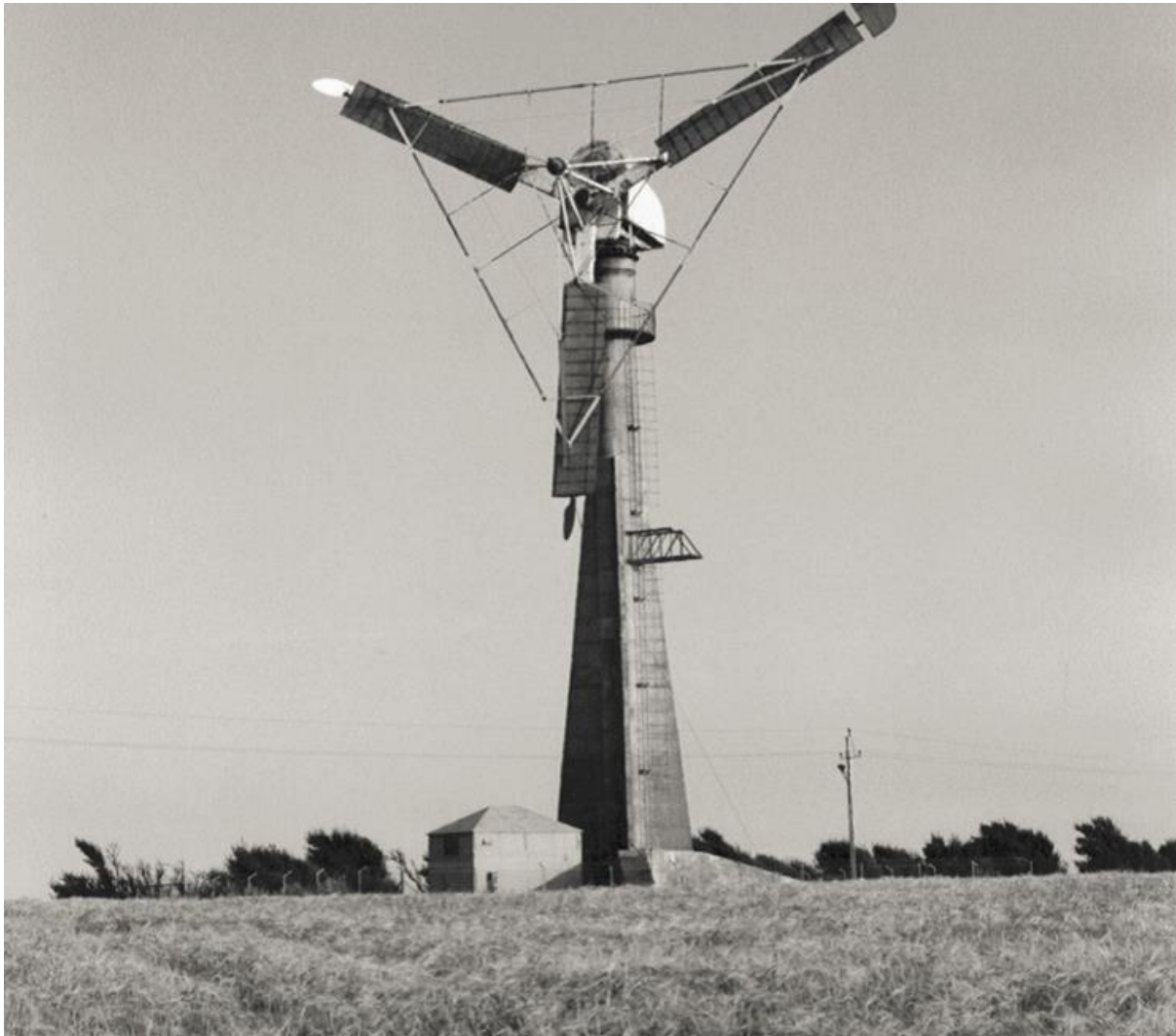
Figure 8: Danish Gedser wind turbine (rotor diameter 24 m, rated power 200 kW), 1957 (Hau, 2006, p. 41)
