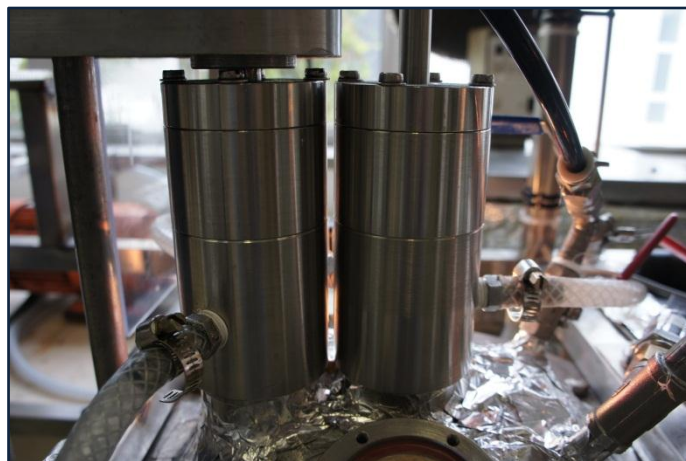
Figure 22 - Mechanical seal housings installed on the top dome of the pressure vessel
