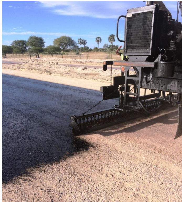
Figure 2-50: Application of prime binder to base
