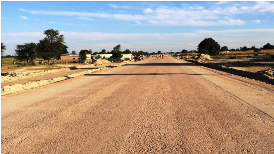
Figure 2-46: Compacted base layer before prime application
