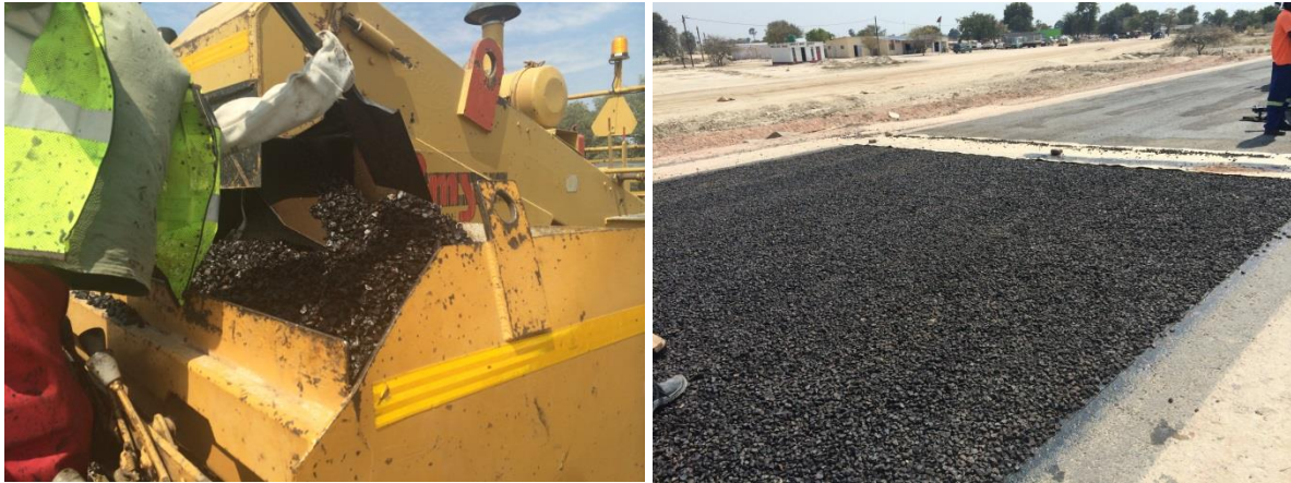
Figure 2-47: A and B: Application of pre-coated aggregate
