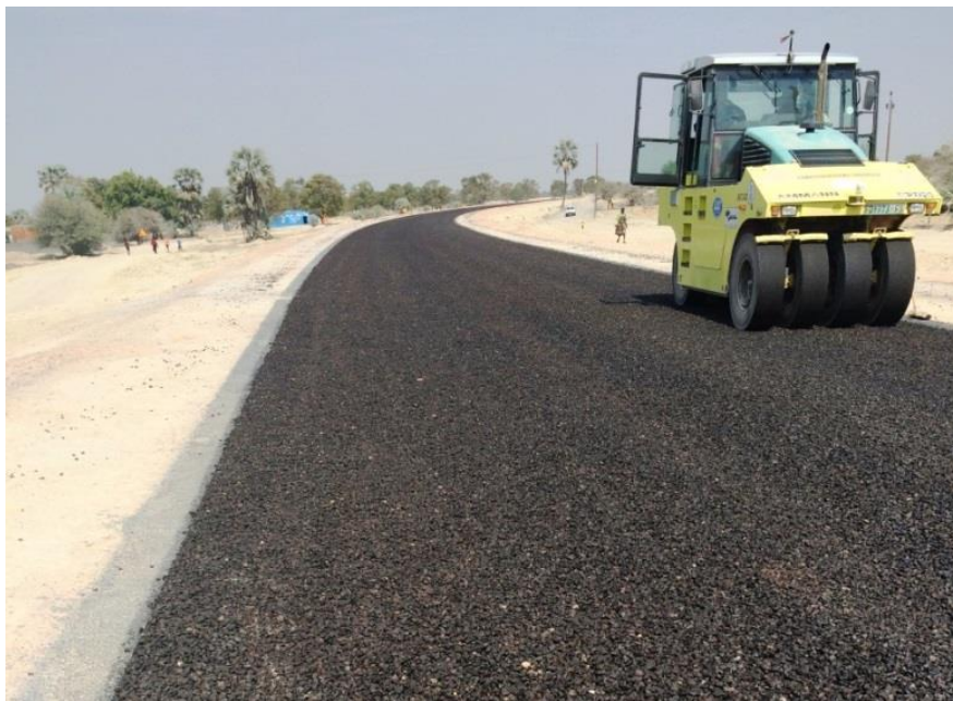
Figure 2-48: Rolling of surface after application
