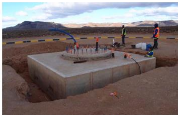
Photo 5: Completed MeerKAT Foundation after stripping of formwork
