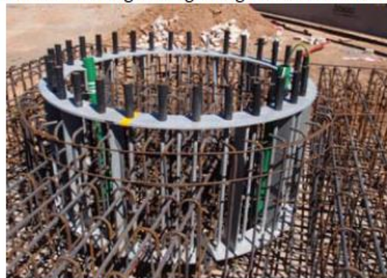
Photo 4: Pile Cap Reinforcement incorporating Bolt Assembly Cage
