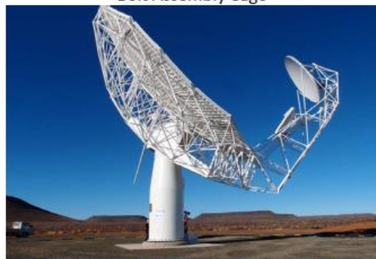
Photo 7: MeerKAT Antenna on a Foundation
