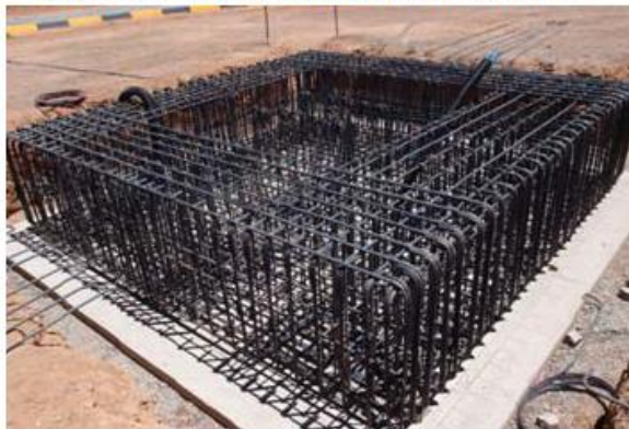
Photo 3: Pile Cap Reinforcement
