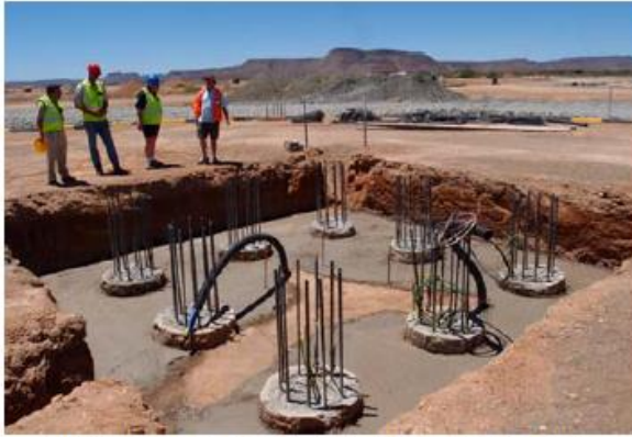
Photo 1: MeerKAT Antenna Foundation Piles
