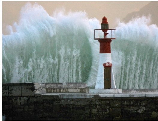
Figure 1.1.2: Photo of a large wave slamming against the breakwater at Kalk Bay Harbour. [Source: http://hqworld.net/gallery/details.php?image_id=23677&sessionid=f0feb15c9f8403838e9ff02ae3c3d692 ]
