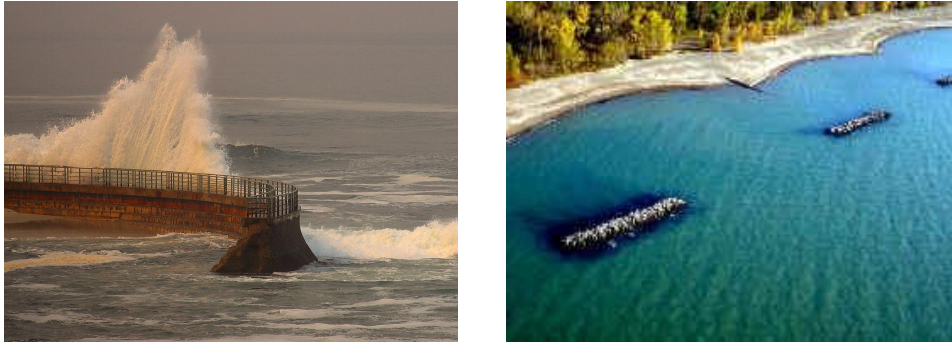
Figure 1.1.1: Examples of coastal defence structures – a seawall on the left and breakwaters on the right. [Source: http://www.studyblue.com/notes/note/n/coastal-protection-measures-hard-engineering/deck/269414 ]
