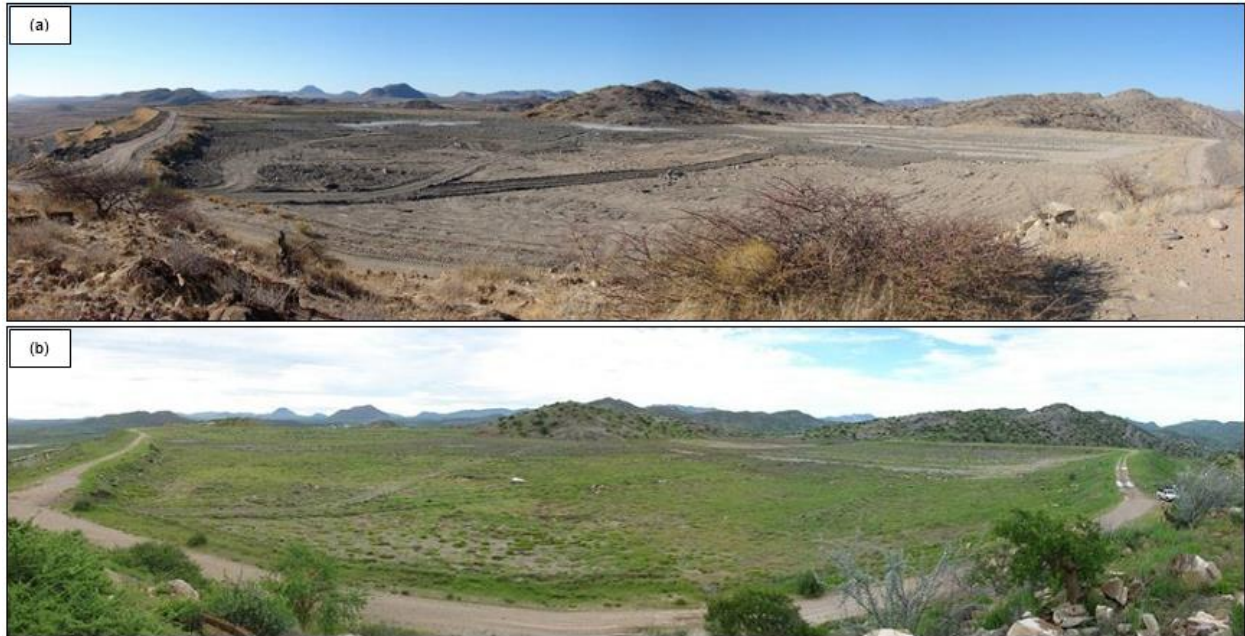
Figure 1.4 Comparison of the top of the first tailings storage facility (TSF1) (a) directly after capping in January 2005 and (b) in March 2009 following a few years of rehabilitation. Source: author
