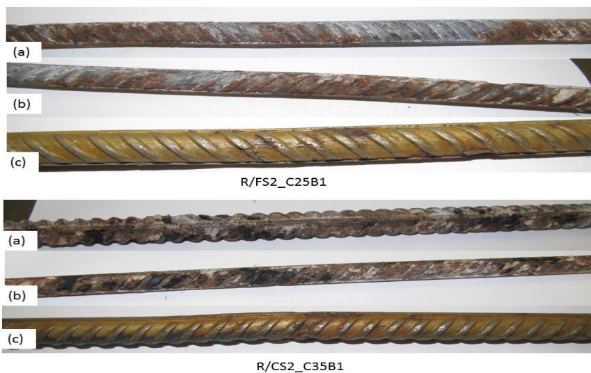
Figure C.13: Corrosion in steel bars in Series One
