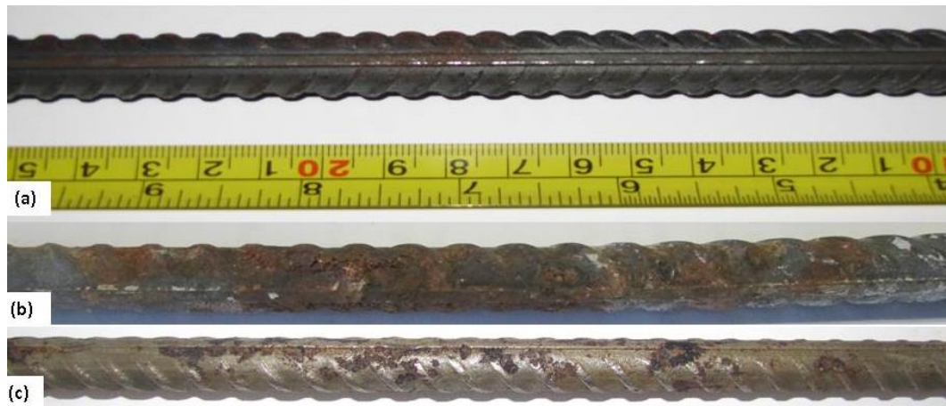
Figure 7.19: Corrosion inspection by destruction method (a) virgin steel (b) R/FS31_C15D5 steel before cleaning and (c) R/FS31_C15D5 steel after cleaning with HCl.
