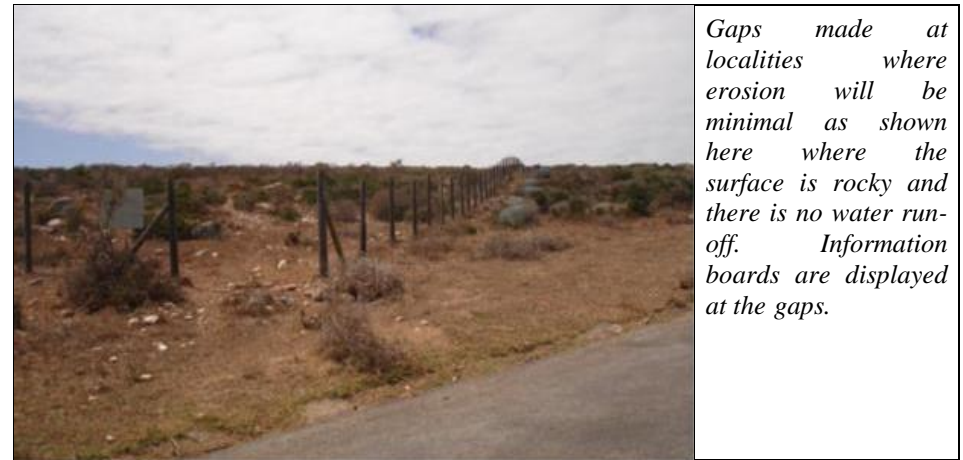
Figure 3.52 New fence with migration gap
