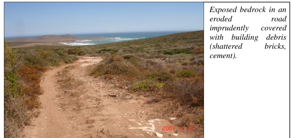
Figure 3.8 Crude rehabilitation of the Plankies Bay road
