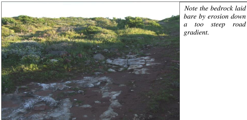
Figure 3.7 Deteriorating unplanned road above Plankies Bay
