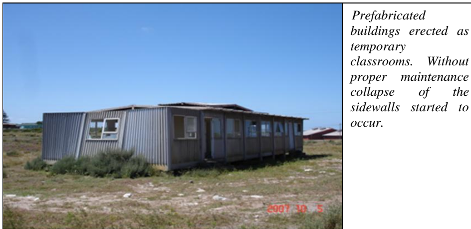
Figure 3.57 Deteriorating prefabricated structure at DMTA shooting range
