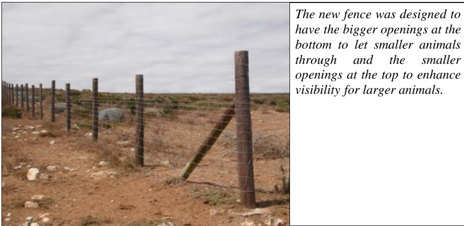
Figure 3.51 New fence stretching from Perlemoen Point to Plankies Bay
