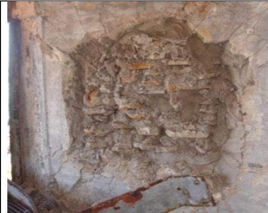
Figure 3.41 Restoration of the wall of a WWII structure wall at Elands Point
