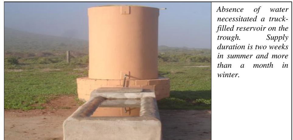
Figure 3.24 New water-trough at South Head
