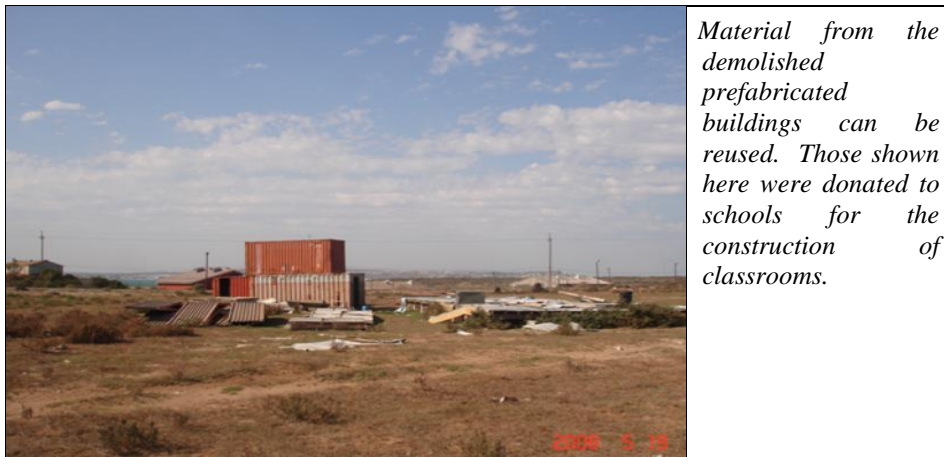
Figure 3.65 Demolishing and removal of prefabricated buildings
