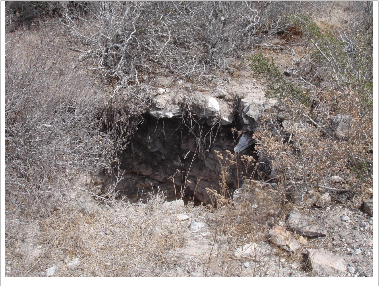
Figure 2.6 Karst-like sinkhole on DMTA
