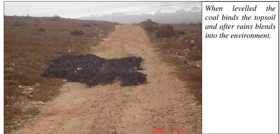
Figure 3.22 Road repair with refuse coal on the road to South Head
