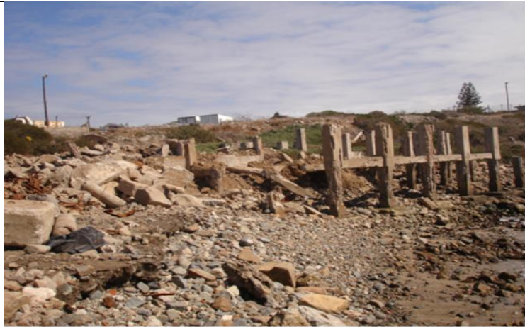
Figure 3.40 Damaged 1930 flensing-platform pillars, Salamander
