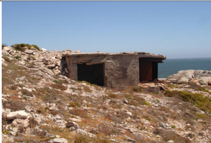
Figure 3.42 Repaired WWII structure at Elands Point
