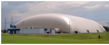
(c) Membrane structures with full gas volumes
