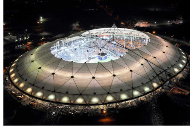
(a) Permanent membrane structures with external pretension
