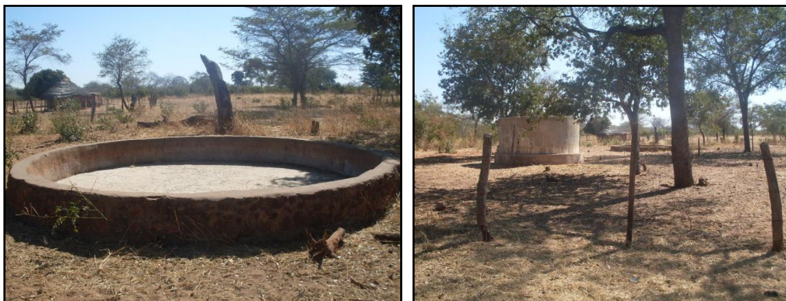
Figure 6-7 Malfunctioning water trough and tank in Monde
