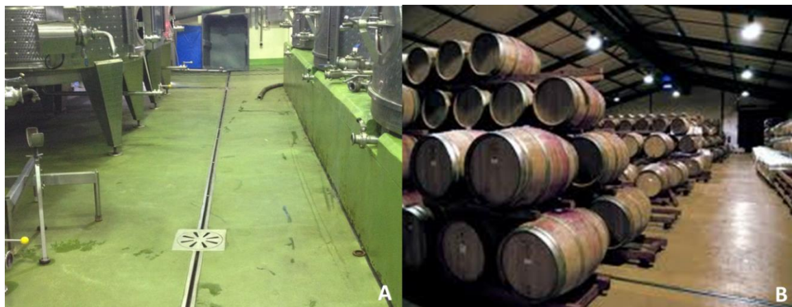
Figure 3.10 Recoated floors of Winery B: A) processing cellar; B) barrel cellar.
