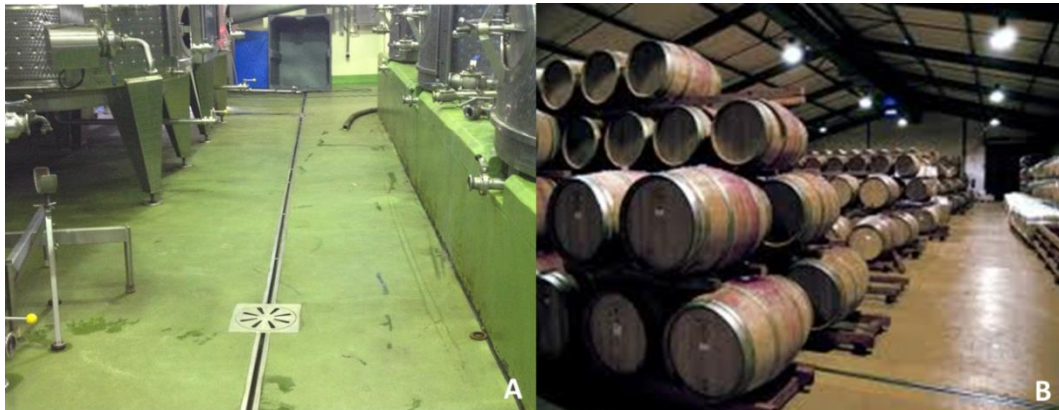
Figure 4.2 Recoated floors of Winery B: A) processing cellar; B) barrel cellar.
