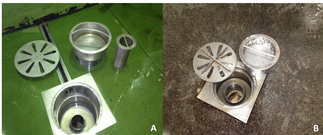
Figure 4.10 A) Double mesh sieves installed in the wastewater drains in Winery B floors. B) Single mesh sieve installed in the wastewater drains Winery A’s winery floors.
