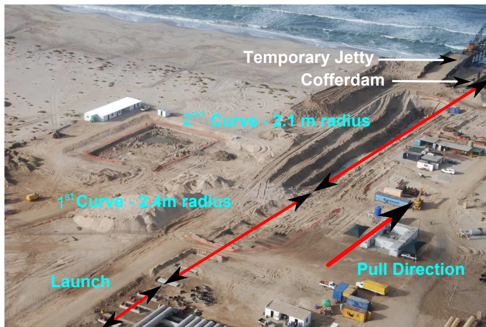
FIGURE 2.9: Trekkopje Pipe Launch Way
