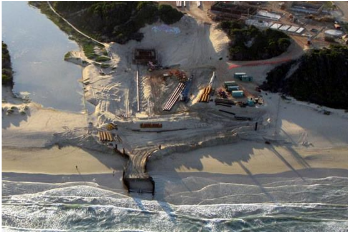
FIGURE 3.5: Mossel Bay Cofferdam Photo During Construction (2011)(Image from Clough Murray & Roberts Marine)
