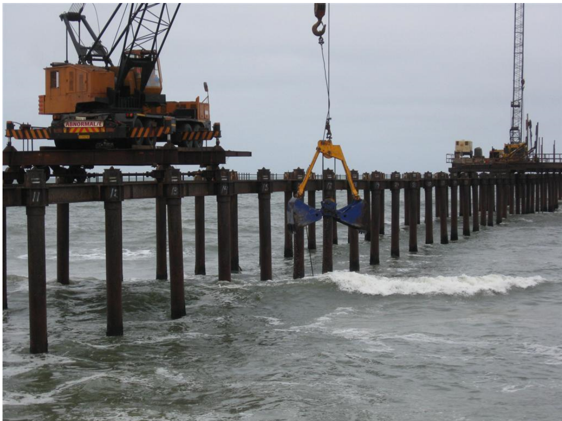
FIGURE 3.2: Trekkopje Cofferdam Photo During Construction (2011)(Image from Clough Murray & Roberts Marine)
