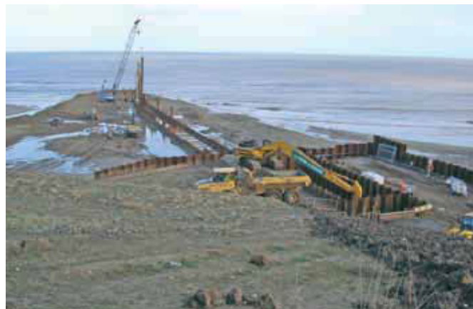
FIGURE 2.18: Langed Cofferdam Construction (Vercruysse and Fitzsimons, 2006)
