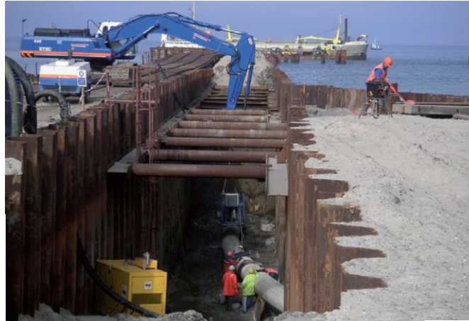
FIGURE 2.21: Balgzand to Bacton tie-in-pit(Boskalis Dredging and Marine Experts, 2012)
