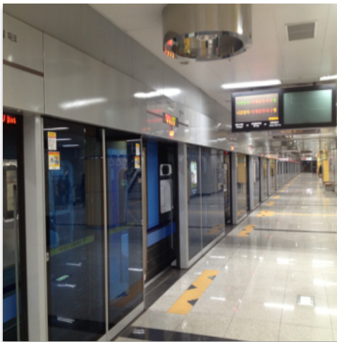
Figure 4.16 Campus town station
