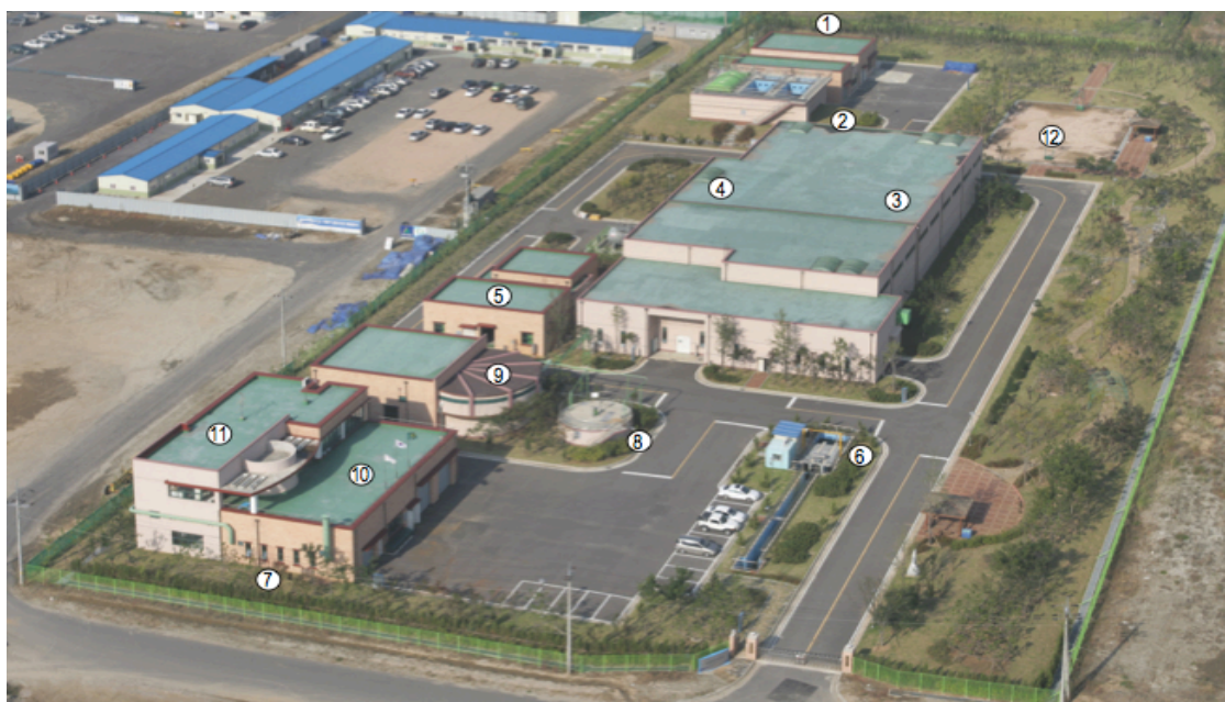
Figure 4.2 Wastewater treatment facilities
