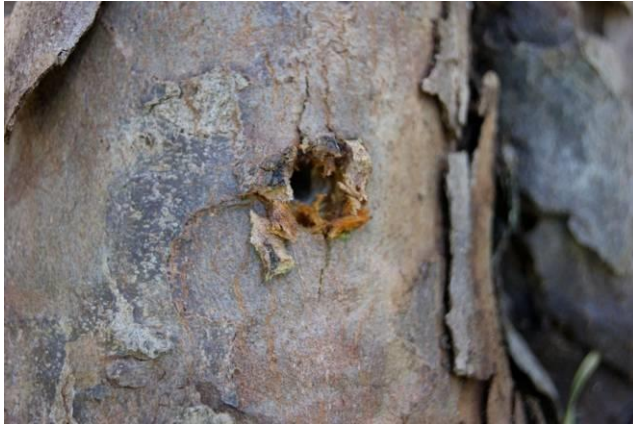
Figure 9: Hole left by borer
