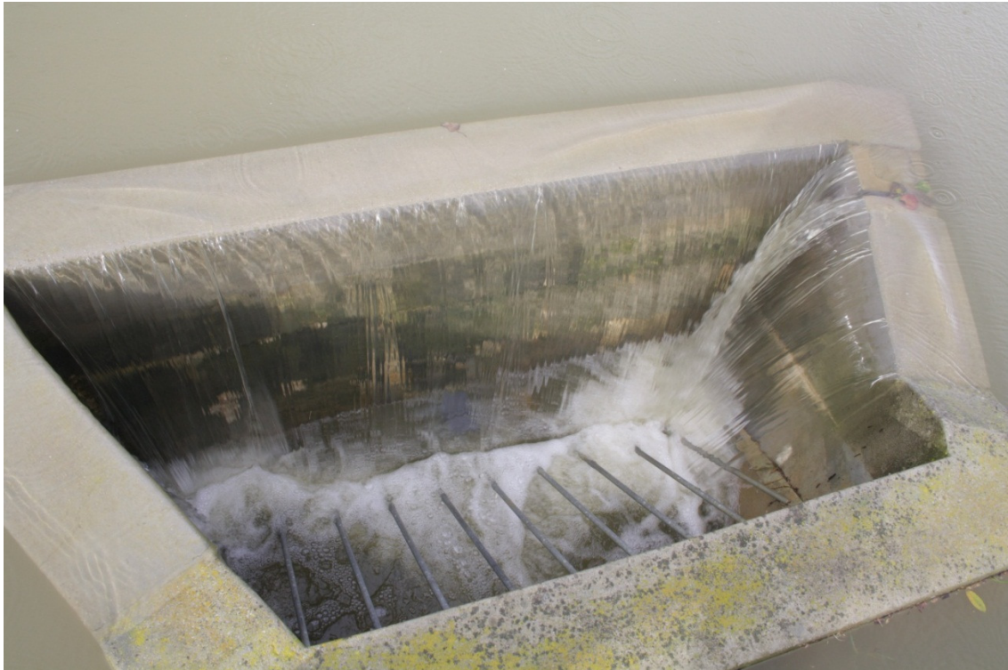
Figure 2.8: Retention pond outlet in Durbanville area
