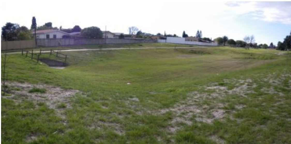
Figure 2.3: Typical detention (dry) pond in the Brackenfell area, Cape Town
