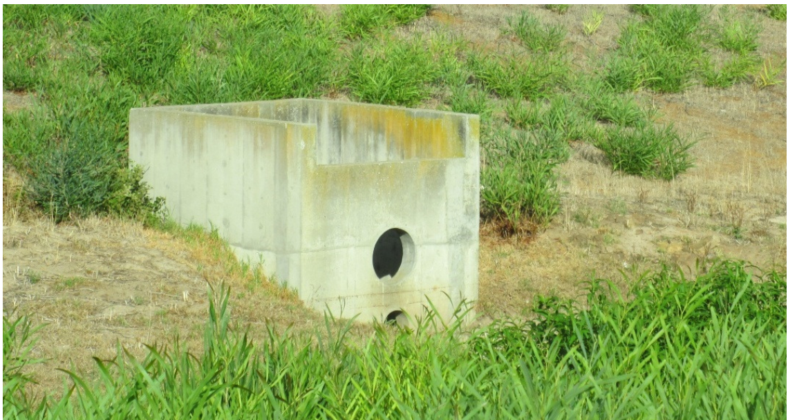
Figure 2.11: Multi-leveled outlet structure in Atlantis
