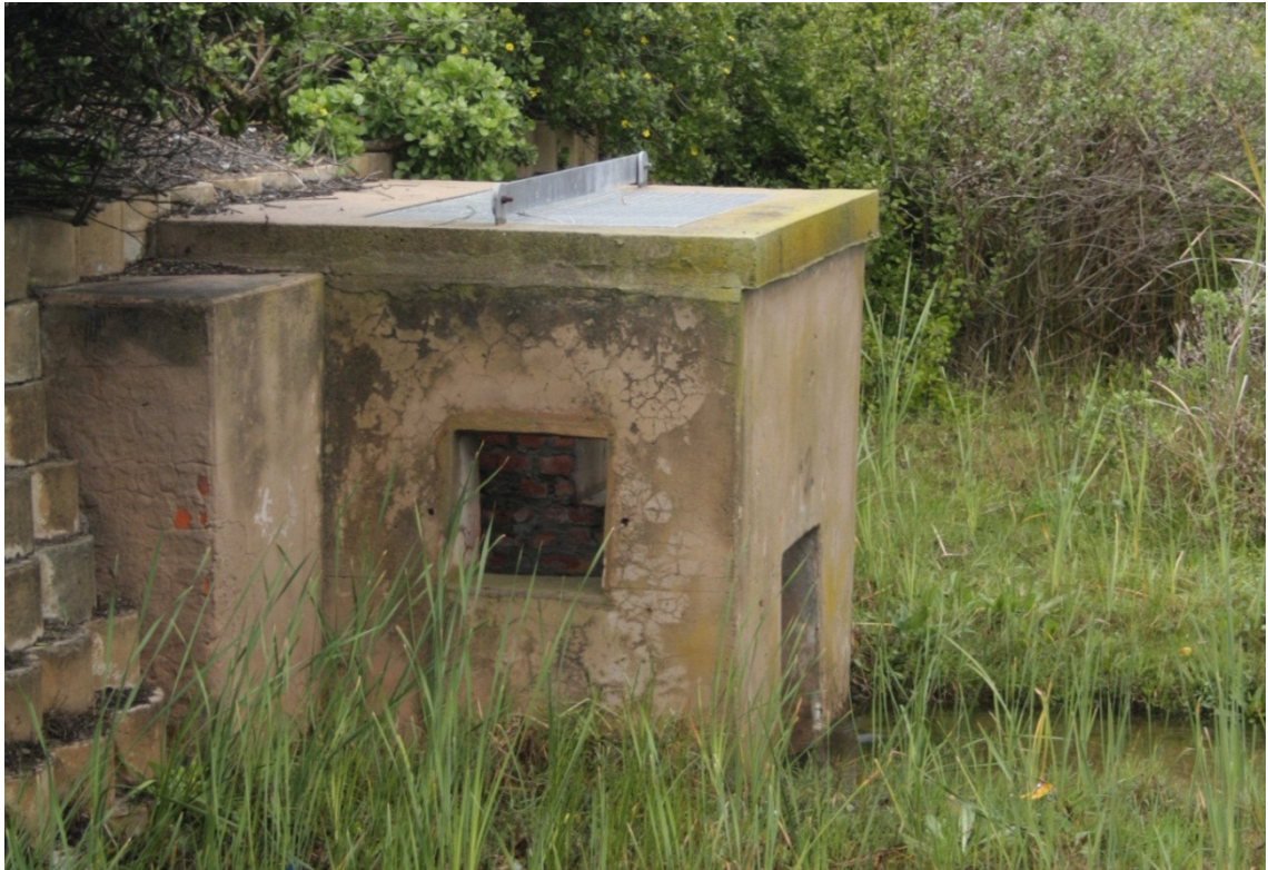
Figure 2.10: Multi-level outlet structure in Sunningdale area, Blaauwberg
