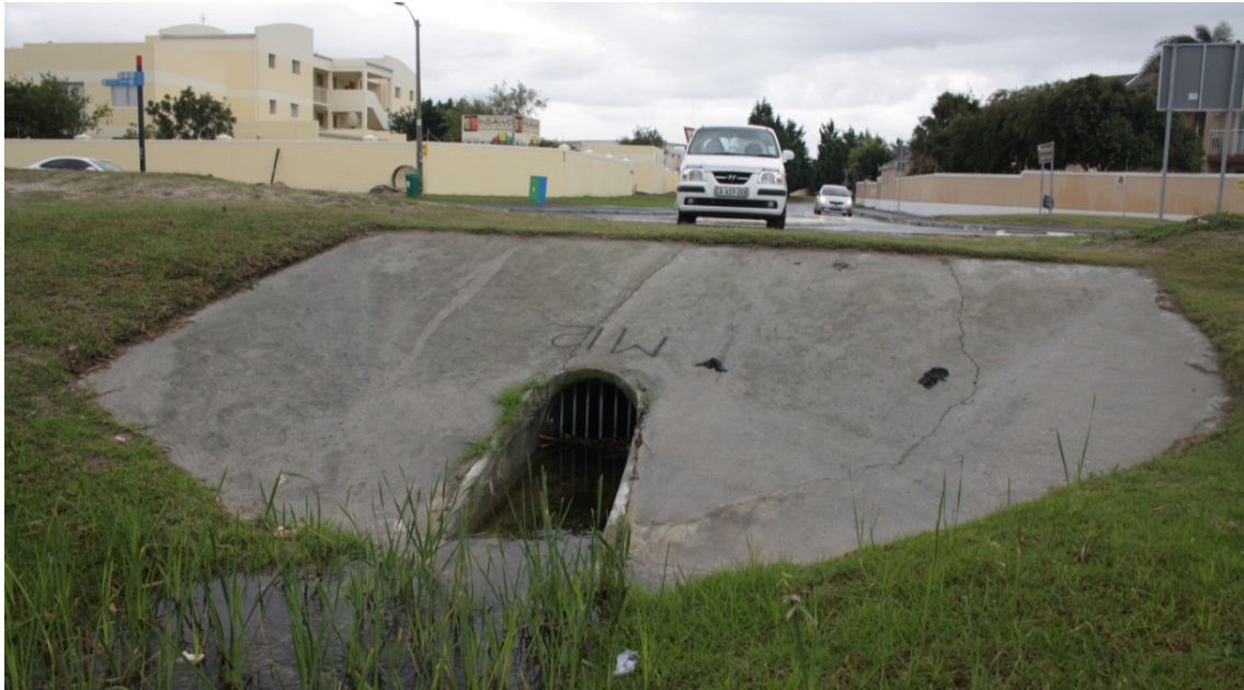
Figure 2.6: Single culvert-type outlet of a detention pond in the Blaauwberg area
