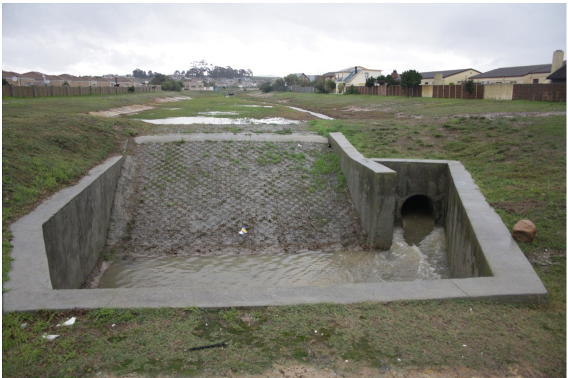
Figure 2.7: Detention pond outlet structure in Kraaifontein area
