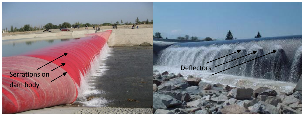
Figure 2.4 Serrations and deflectors on inflatable weir (Brussels, 2006)
