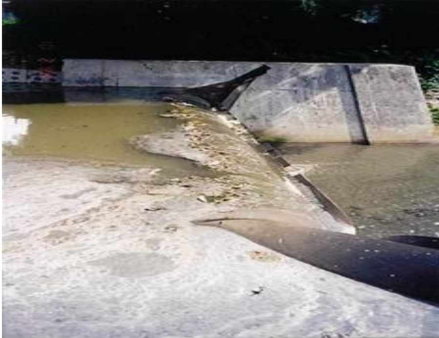
Figure 2.8 V-notch behavior of air filled weir partially filled (Alwan, 1979)
