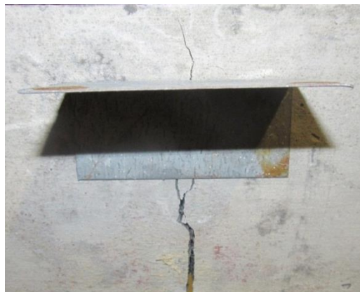
Figure 47: Metal plate for LVDT to press against not affecting crack formation
