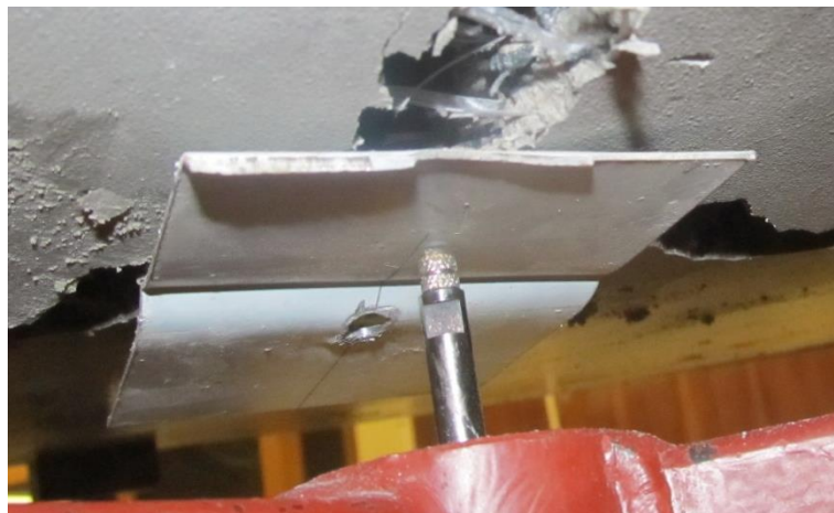
Figure 49: Metal plate preventing LVDT from slipping into cracks
