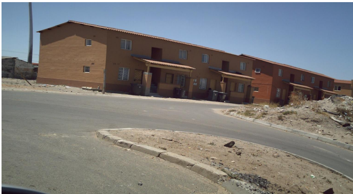
Figure 5: A Completely new block-Gap in-fill for Overflowing Residents.
