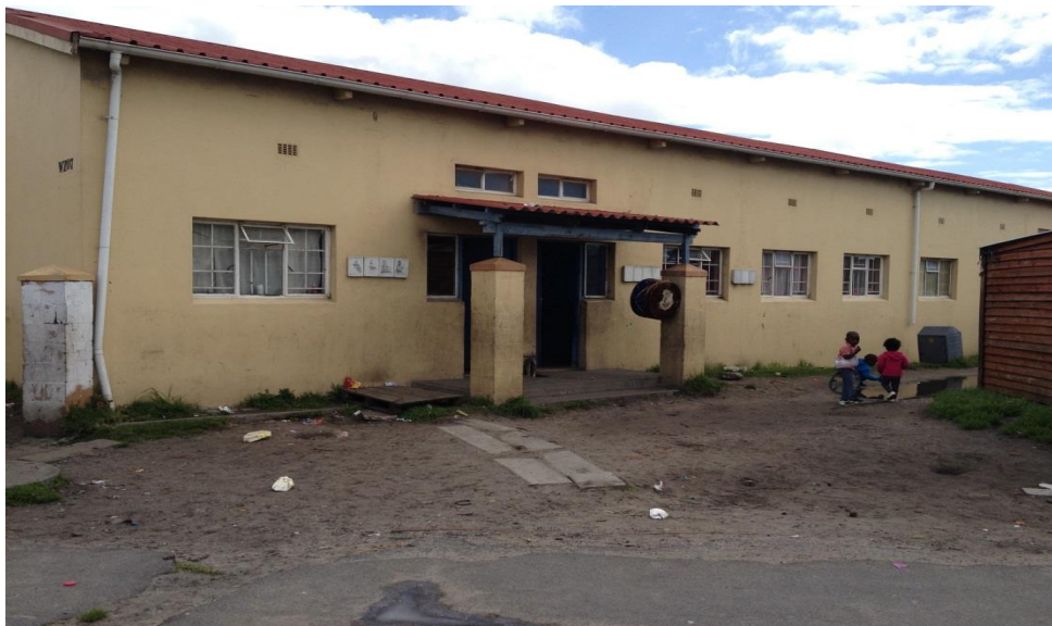
Figure 37: Another housing design for the Langa Hostel Redevelopment Program
