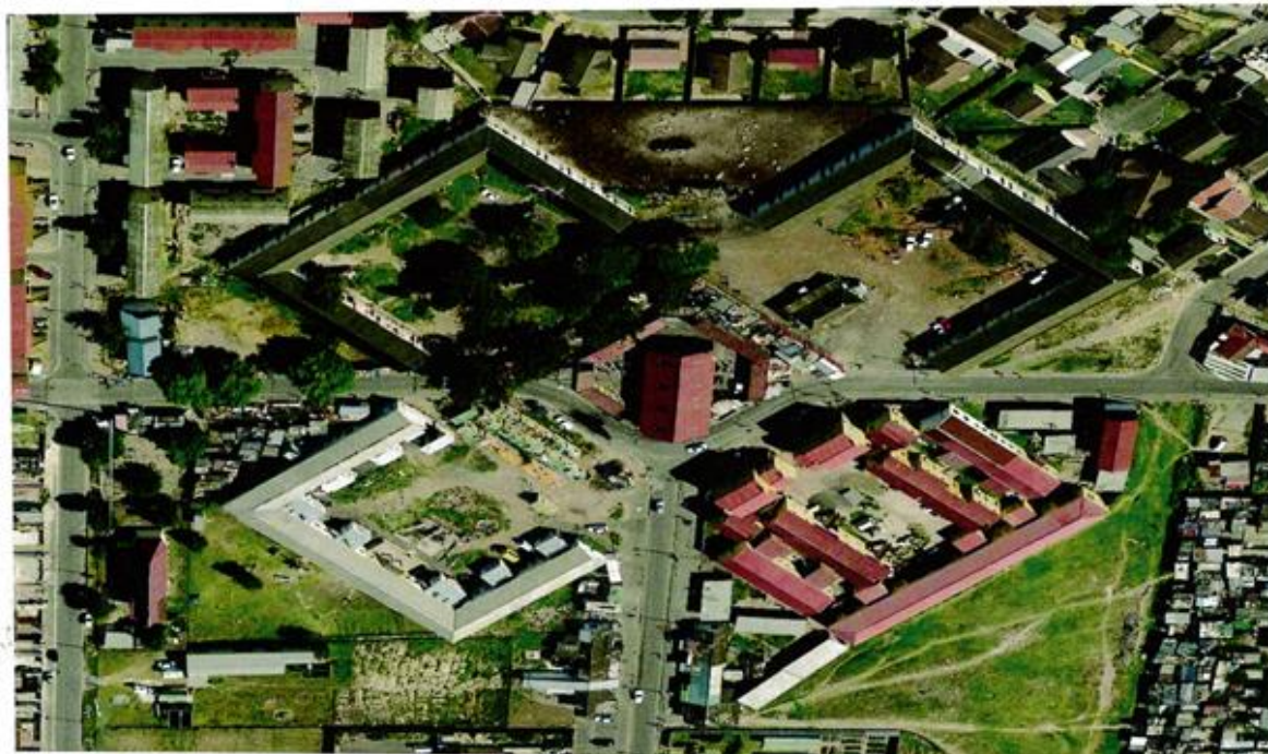
Figure 23: Langa Barracks and Welcome Zenzile Hostel Redevelopment Program [Red roof]
