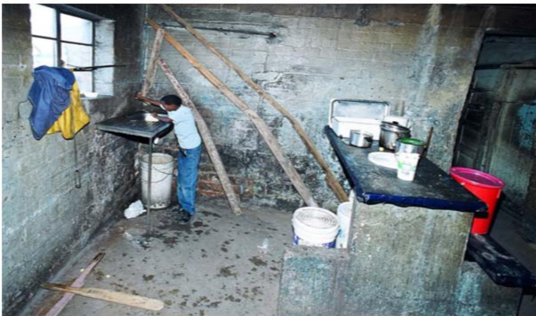
Figure 28: A badly maintained communal cooking and eating space in a hostel in Langa
