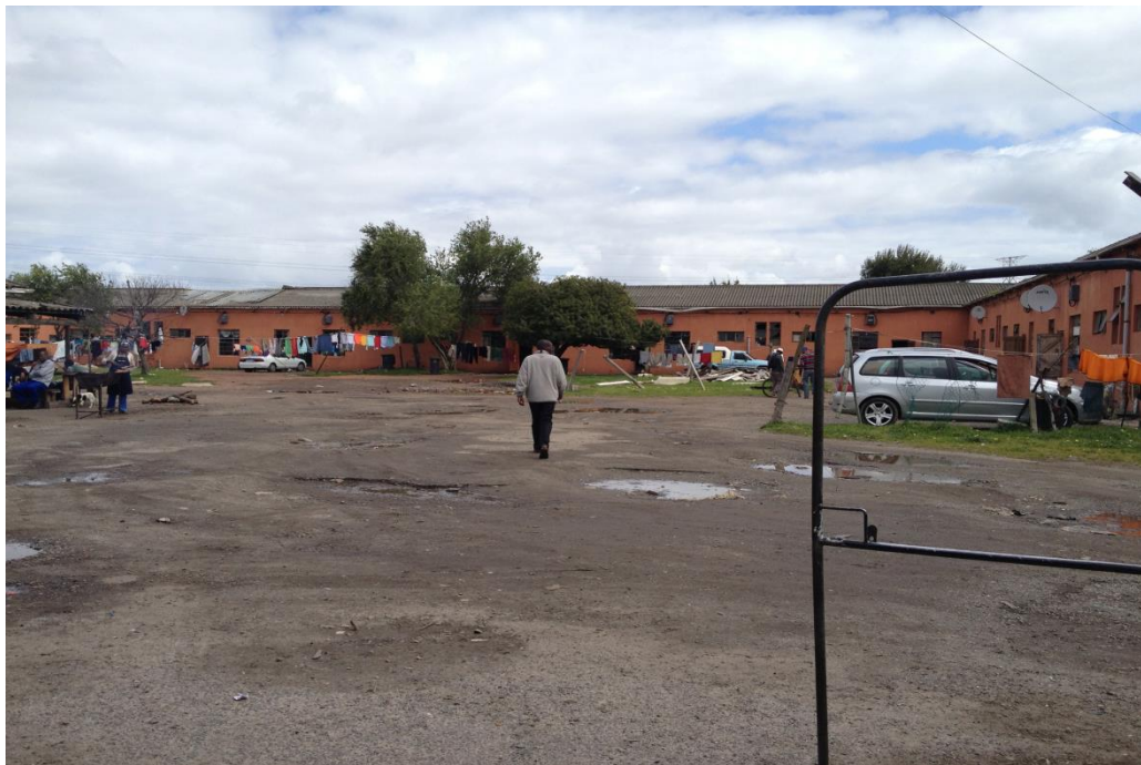
Figure 33: A recently 'renovated' block of the old South Barack
