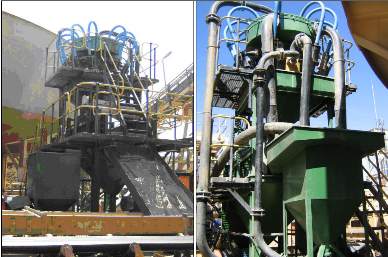
Figure 1-3: The assembled Hi-G Dryer unit at Daberas
