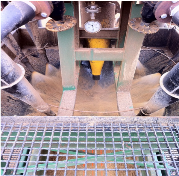
Figure 4-12: The primary cyclone under roping conditions discharging with the cluster cyclones
