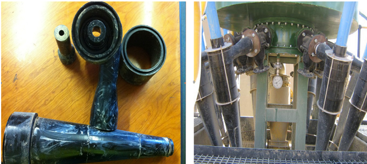
Figure 2-4: One of the cluster cyclones dismantled (left) and the 12 radially mounted cyclones above the Hi-G screen (right)
