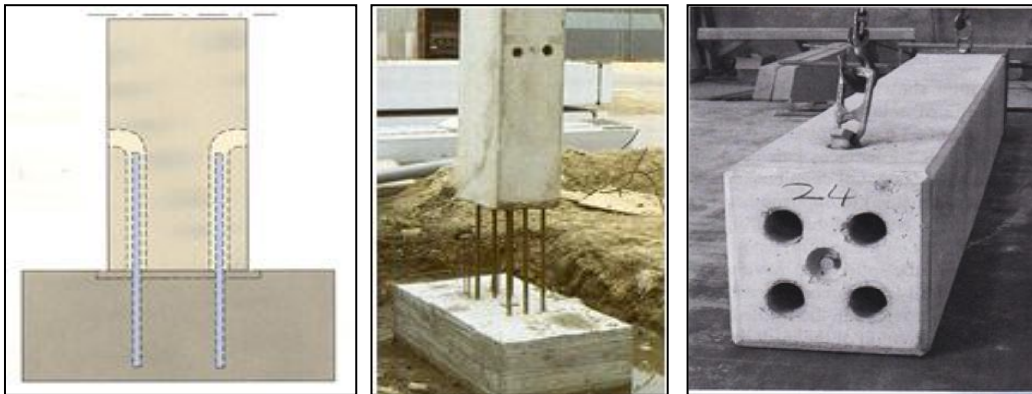
Figure 2.10 - Illustrations of projecting bar connections (Van Acker 1996)
