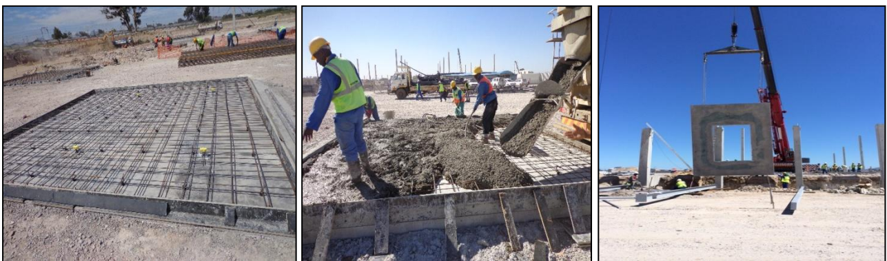
Figure A.9 - Different steps in tilt-up construction (Group 5, 2014)
