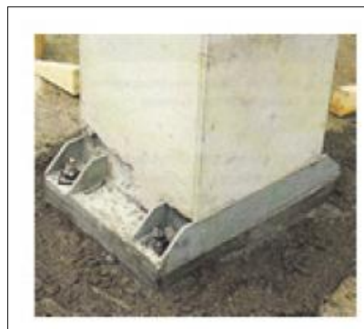
Figure 2.9 - Some illustrations of precast concrete baseplate (The Shockey Precast Group 2001)
