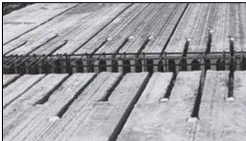
Figure 2.26 – Openings created for reinforcement in hollow core slabs (Nakano, Matsuzaki 1996)
