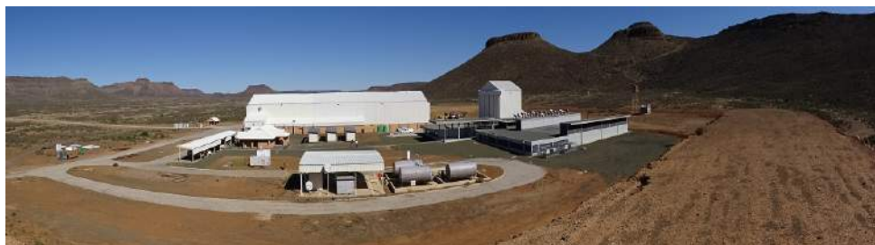
(a) Transmitting side of the Berm.
