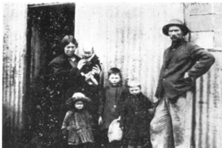
Figure 38: House and family of a white diamond digger
