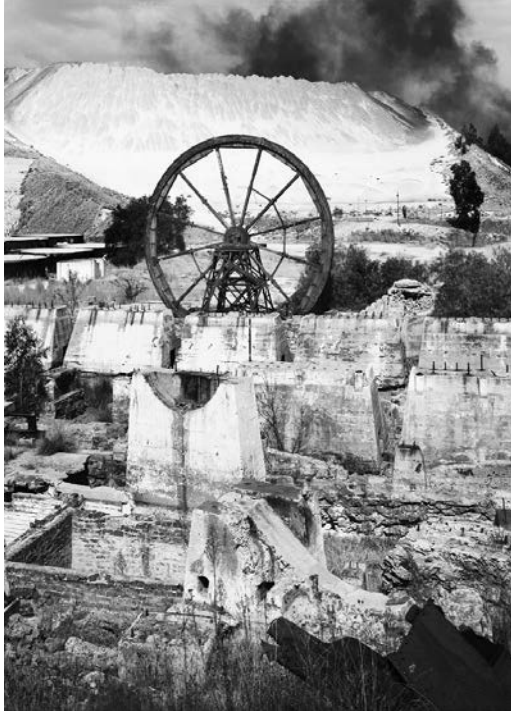
Figure 4: David Goldblatt (1966) Old mill foundations, tailing wheel and sand dump, Witwatersrand Deep Gold Mine, Germiston.
